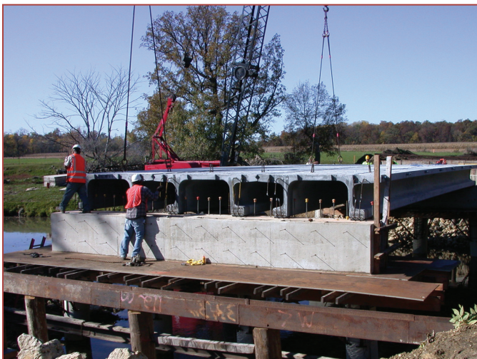
Construction using the second-generation pi-girders (cast with an integral deck and enhanced wear surface durability)
