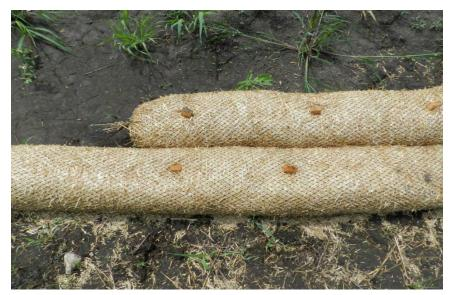
Ditch check showing wood stakes at correct spacing and controls overlapped.
