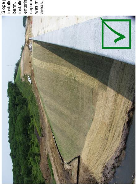
Slope protection was installed on this bridge berm. Silt fence was also installed to control silt from entering the river and to separate the area that was matted from disturbed
