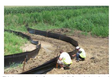
This is an example of a second silt fence being placed as a replacement where the existing fence was blown out. To be more effective, the new fence should have been installed downstream of the existing fence.
