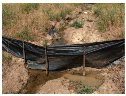
This ditch check has been undermined and should be removed.
