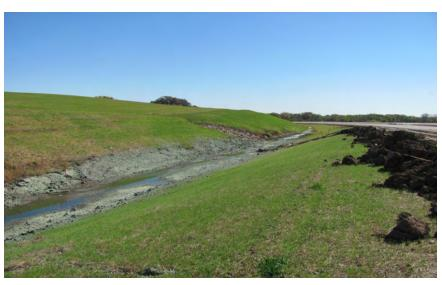
An example of an area where the contractor used hydraulic seeding and mulching to reseed an area that was wet and would have been difficult to access.
