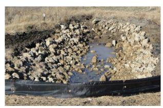
Riprap has been placed around this inlet to prevent erosion. Silt fence has been placed to prevent sediment from entering the inlet.
