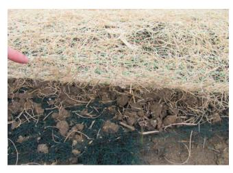
This detail and photo show installation of TRM, which includes TRM, topsoil, and special ditch control.
