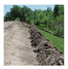
Vegetated buffer used with silt fence and topsoil berm.
