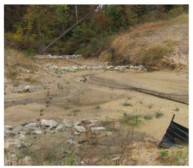
This silt basin's capacity has been reduced by more than 50% and requires clean-out.
