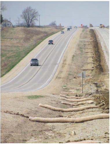
Here logs worked well as ditch checks in a shallow median.
