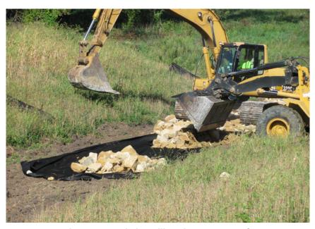
A contractor is installing riprap on top of engineering fabric to create a rock ditch.
