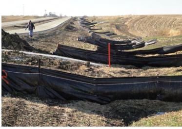
This photo shows a chain of silt fence ditch checks installed to slow velocity of water and collect sediment from flowing downstream.
