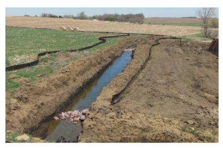
Temporary stream diversion showing a diversion channel and upland sediment controls.
