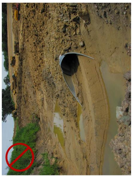
This pipe culvert has no controls around it. A silt basin and silt fence are recommended controls for this area.
