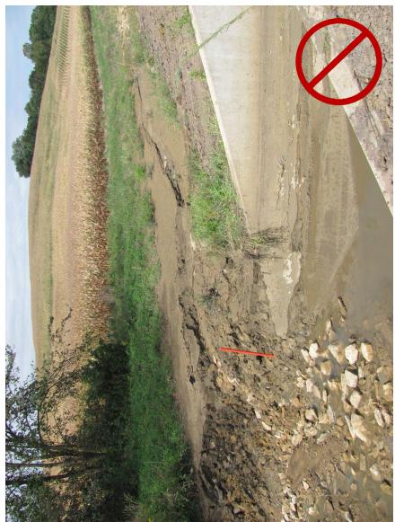
This photo was taken shortly after the outlet end of a box culvert was cleaned out. Based on the silt still remaining in the ditch and the dirt line on the culvert, it's estimated about two feet of silt was removed. The entire site should be reviewed to find what structural controls are needed and areas that should be stabilized. A single silt fence will not prevent recurrence.
