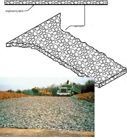
A stabilized construction entrance is designed to minimize tracking of sediment from the site by vehicles and equipment.
