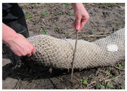
Devices should be installed with proper staking. This photo shows <u>improper</u> staking using a metal nail.
