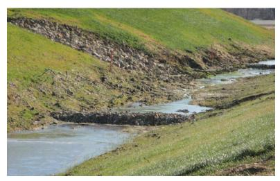
The end of a rock check dam should extend up into the side of the slope. The low point should not be at the side; otherwise water will just flow around the ditch check and erode the slope.
