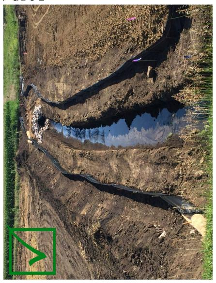
This shows a good example of a temporary stream diversion installed per EW-402.
