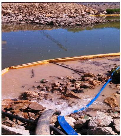
Silt curtain used as a separation barrier to keep turbid water from entering the flowing water body. Additionally, the dewatering hose is outletted onto rock.
