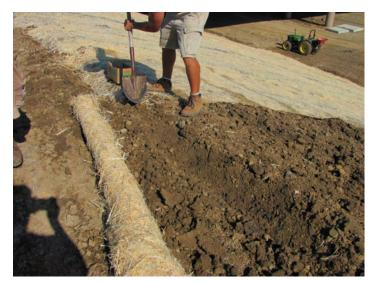
It is important to ensure that the contractor installs the slope protection properly – this includes using anchor slots at the top of the slope protection to ensure flows do not travel underneath.
