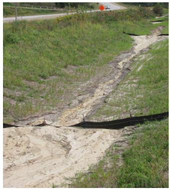
Silt fence ditch checks at capacity require removal and replacement or clean-out.
