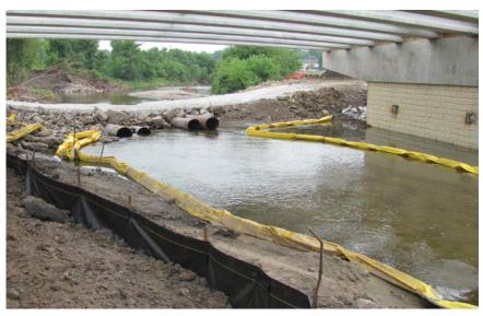
A temporary stream crossing was constructed by the contractor to allow for access to both sides of the creek. When a temporary stream crossing is used, it should be completed according to EW-401.
