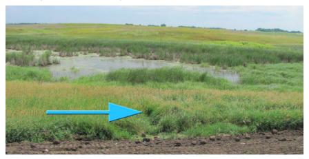
Existing vegetation used as vegetated buffer in conjunction with silt fence (indicated by blue arrow) to protect a wetland.
