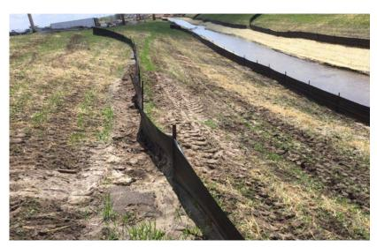
This photo shows a silt fence that was cleaned out. However, the removed silt was incorrectly placed in front of the silt fence.
