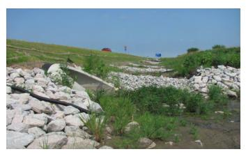
This photo shows rock ditch checks, silt basins, silt fence, logs, and temporary vegetation used to protect a discharge point.
