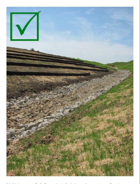
Multiple rows of silt fence installed along the contour of a slope. Due to the ditch grades, a rock ditch was installed to prevent erosion in the ditch. The backslope was also seeded prior to the road embankment being completed.
