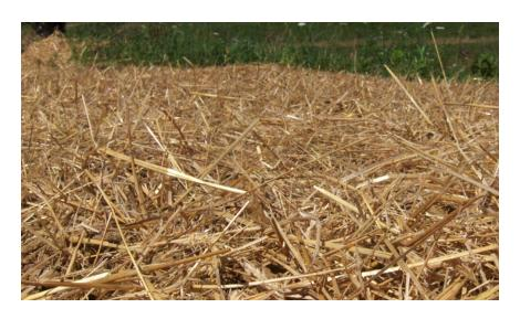
Mulch should be applied evenly without large piles or bare spots. It should be anchored into the soil.
