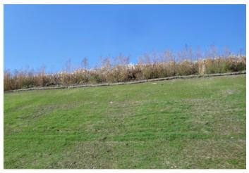
Devices installed at the top of a slope to help vegetation get established on the slope.
