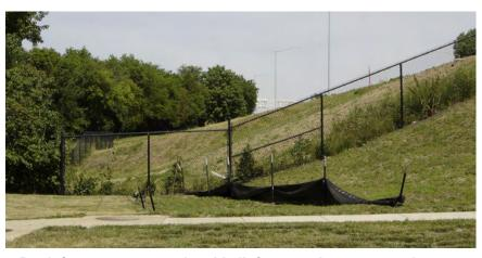
Don't forget to remove the old silt fence and posts once the area has reached a density of 70%. Posts should be pulled and silt fence should be cut off at ground level or completely removed.
