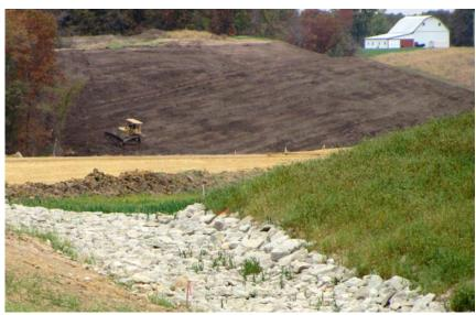
Topsoil was stripped and stockpiled and is shown being respread in the background.
