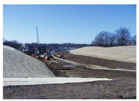
Slope protection slows run-off and keeps the soil moist while seed germinates.
