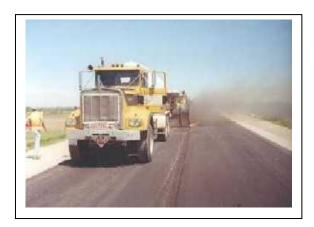
The process is typically used in situations where the existing pavement has surface irregularities, such as minor rutting, oxidation or raveling, but remains structurally sound.
