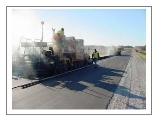
Increasing plant mix temperature, covering hauling units, minimizing haul length, and shortening windrows in front of pickup machines can all minimize the effects of the environment on HMA paving.
