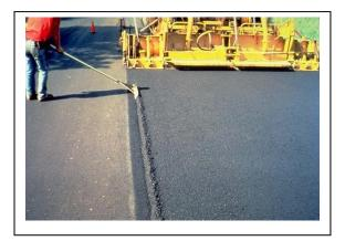
majority of the breakdown roller is being supported by the cold side of the joint.
