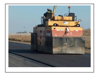
Intermediate rolling is commonly seen on interstate and higher volume primary paving projects, which typically use stiffer mixes and higher crushed aggregate contents.
