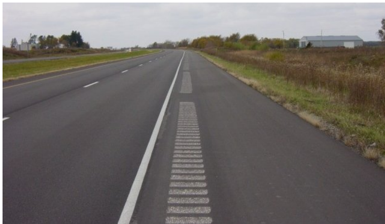
Figure 3: Gapped shoulder rumble strip pattern.
