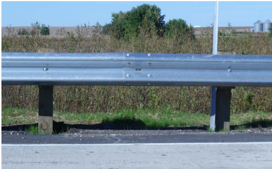
Figure 2: Steel beam guardrail example.
