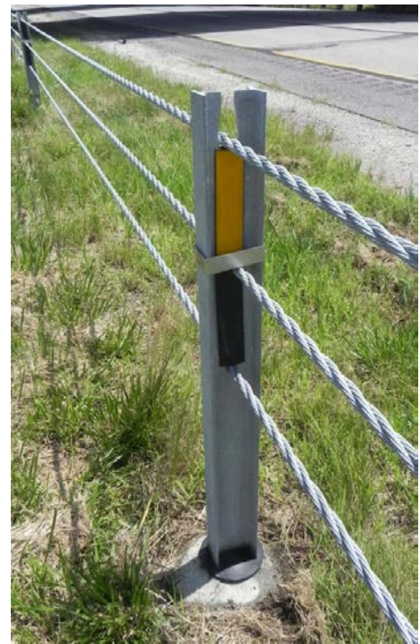
Figure 1: High-tension cable guardrail example.
