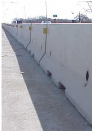
**Figure 2:** Temporary concrete barrier rail example.
