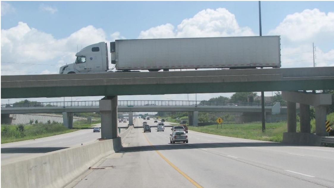
**Figure 1:** Permanent concrete barrier rail example.
