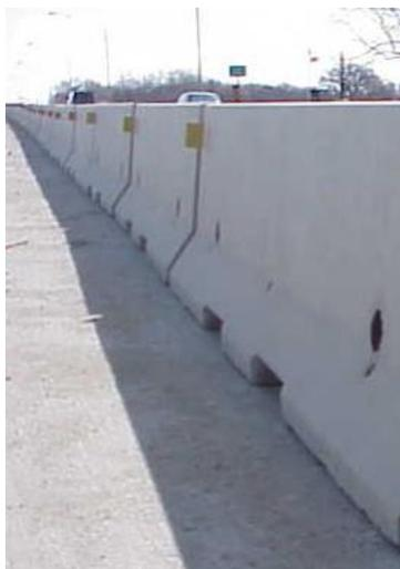
**Figure 2:** Temporary concrete barrier rail example.
