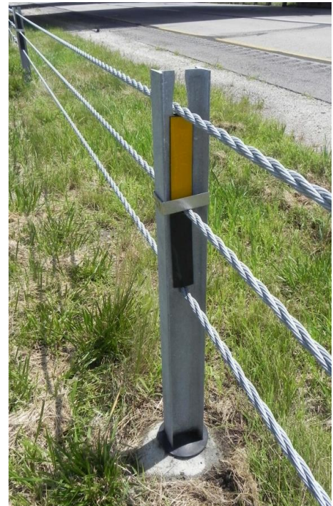
High tension cable guardrail example
