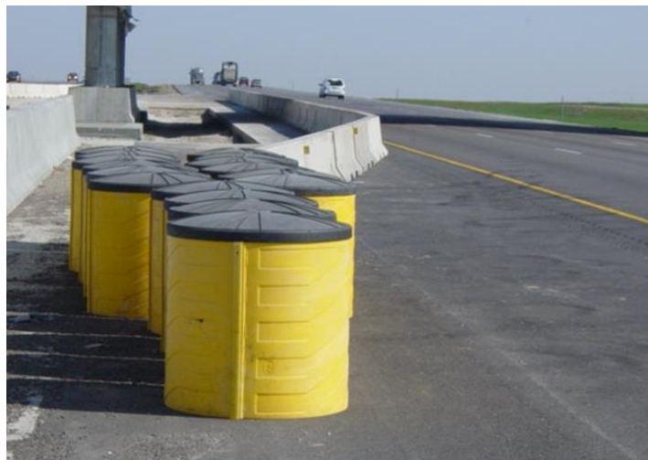
Figure 2: Sand filled barrel arrays are adaptable to many types of obstacles.
