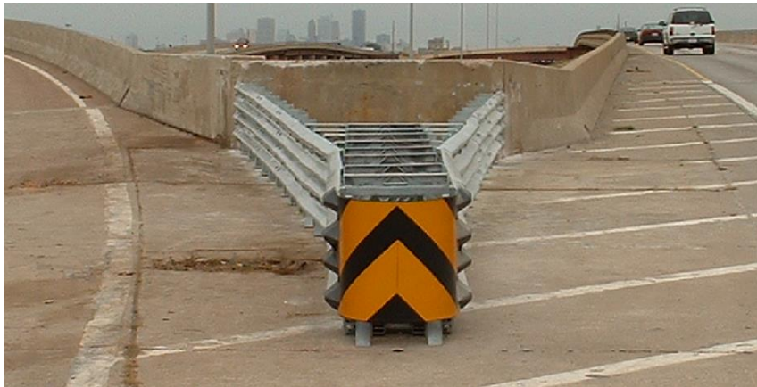
Figure 5: A crash cushion shielding a gore area.
