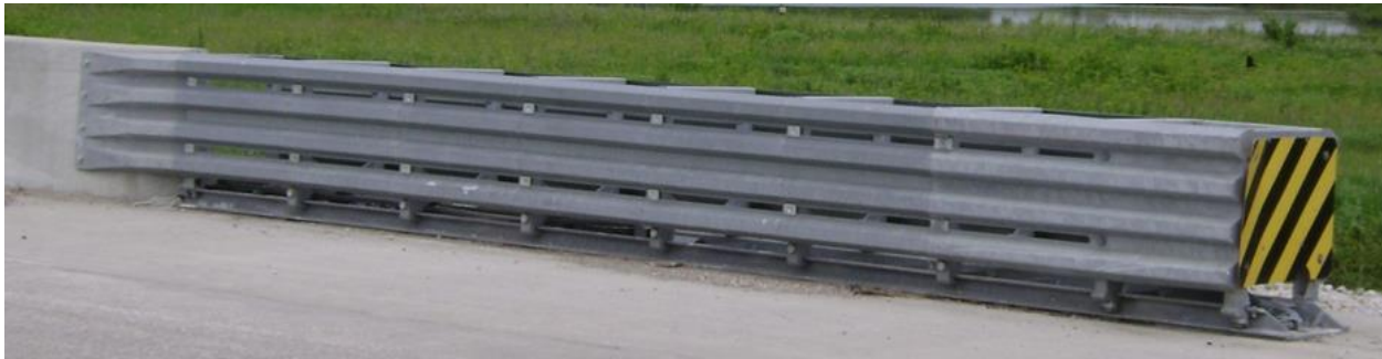
Figure 1: A typical crash cushion.
