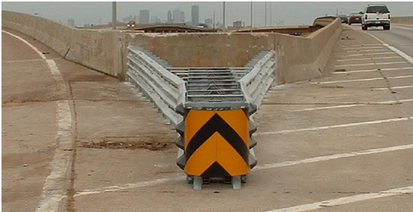
Figure 5: A crash cushion shielding a gore area.
