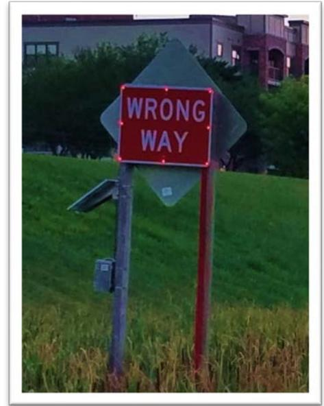
*Flashing wrong-way sign triggered by sensors that detect vehicle entering from the wrong direction.*
