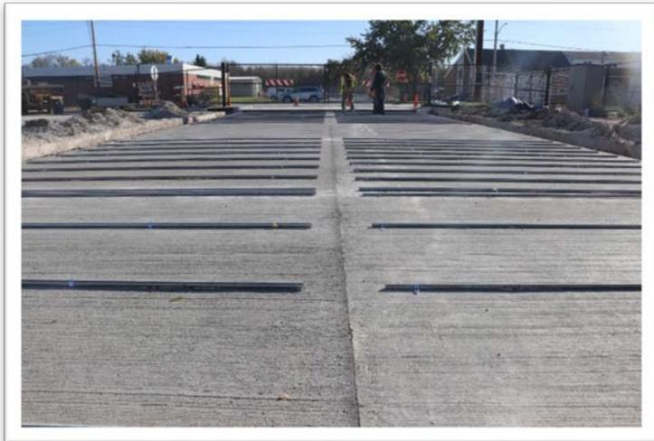
*This photo shows electrodes being installed before the electrically conductive layer was poured.*
