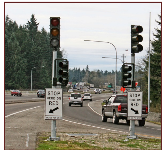
Signals located on on-ramps are interconnected and meter the traffic flow based on mainline congestion throughout the system.
