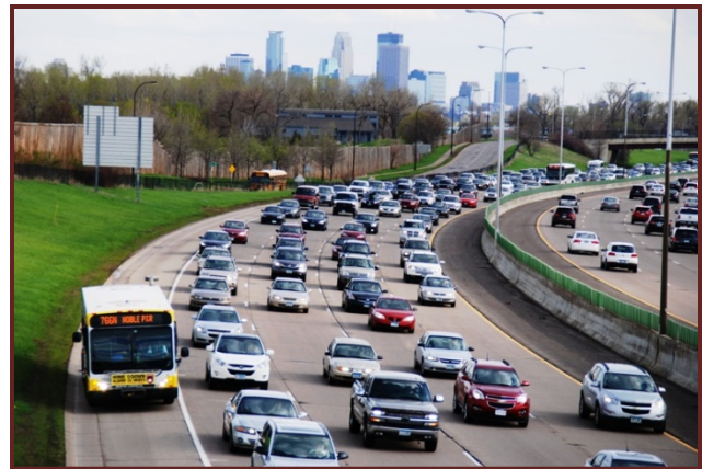
Becoming commonplace in urban areas, bus-on-shoulder operations utilize roadway shoulders during peak commuter periods or during incidents to improve transit reliability.
