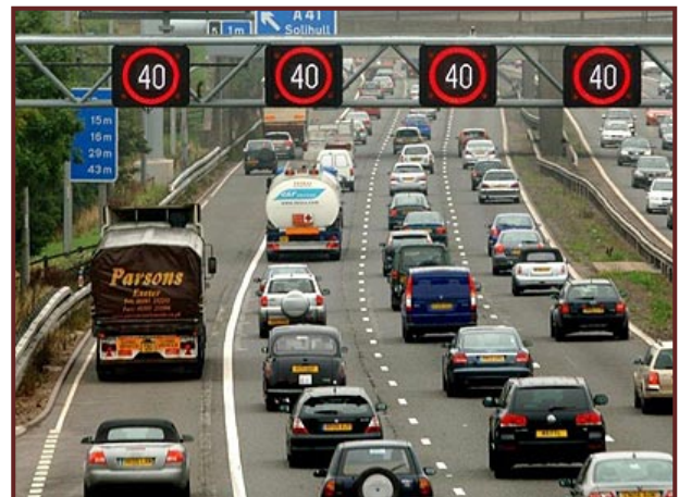
Managed Motorways, a common strategy in the United Kingdom, utilizes traffic flow controls and peak-period shoulder operations to maximize throughput and safety.
