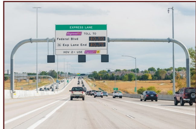
The Express Lane Concept would provide a continuous express lane(s) adjacent to the general lanes and separated by a buffer.
