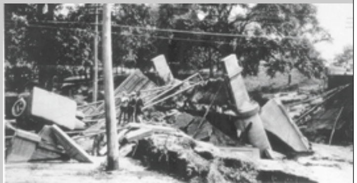
The Squaw Creek bridge on Lincoln Way in Ames, new in 1908, collapsed following the flood of June 3, 1918. A flood earlier in the month weakened the structure and it collapsed as the Goddard family car crossed it. The occupants of the car were not seriously injured and were rescued with ropes and ladders.
