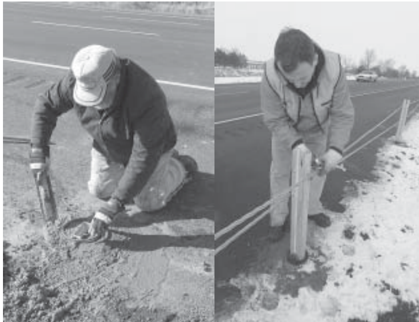
Contractors install the cable barrier on I-35 near Ankeny.
