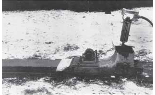
First prototype slipform paver, circa 1947
