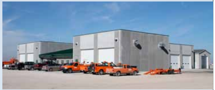
The new Rockwell City maintenance garage will serve the needs of the Iowa DOT for decades to come.
