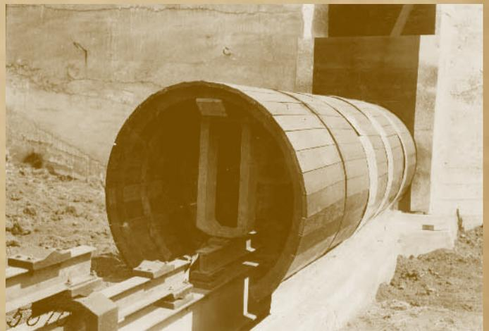
Oblique view of experimental station to determine traffic pressure on culverts in place on highways. Dated between 1910 and 1921 based on the number recorded on the photo.
