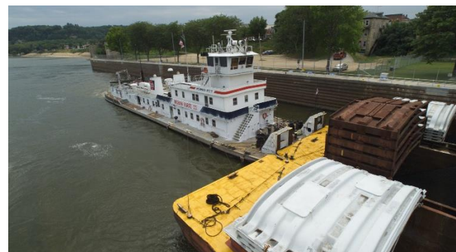
Tug and barges at Lock 12 (Source: Iowa DOT)
