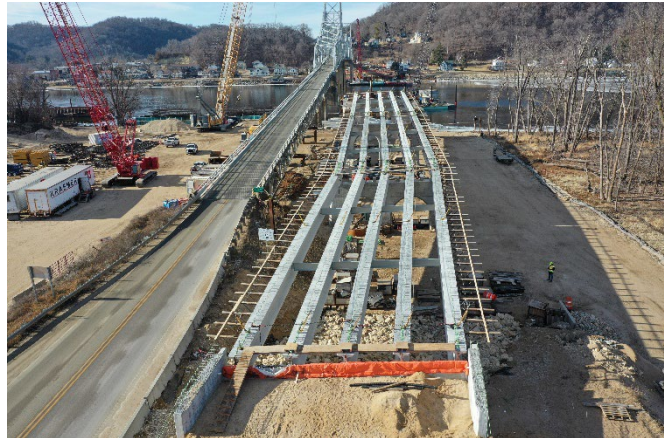
Bridge Beams in Place
