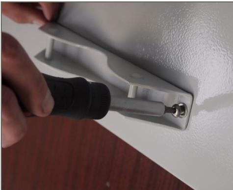
Figure 5: Attaching the banding bracket to the sign
