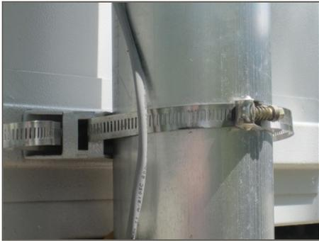
*Figure 7: Sign Secured to a Pole with Banding Strap*
