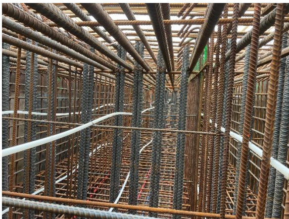
Rebar in Pier 1 Footing
