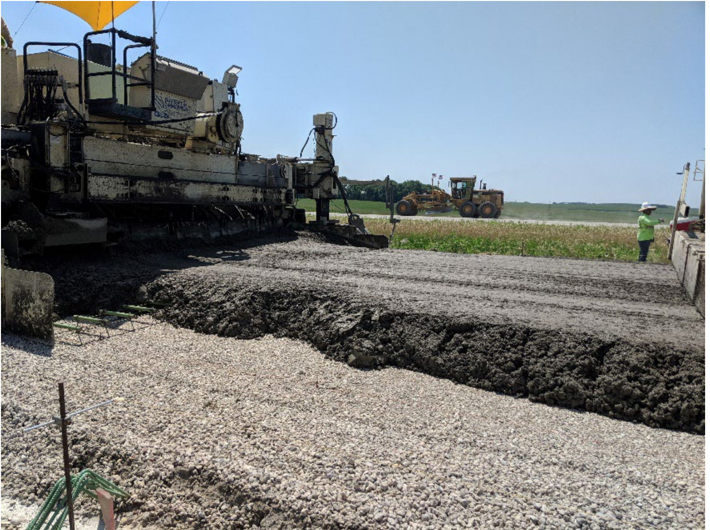
Slipform Paving
