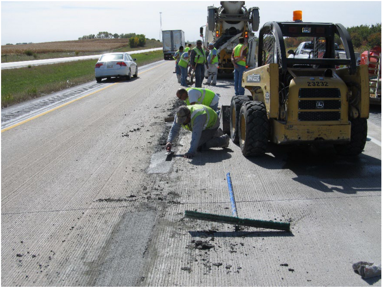
Partial Depth Patching
