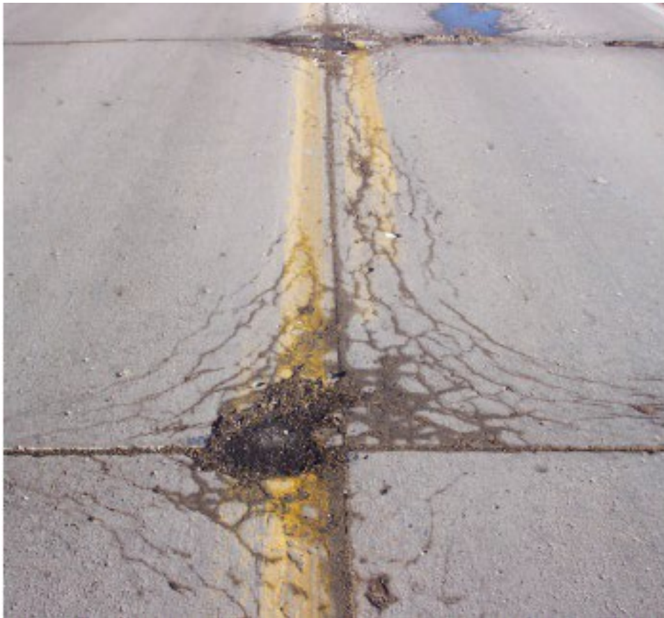
Figure 4-7 D-cracking deterioration
