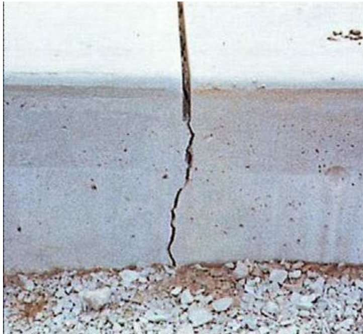
Figure 2-27 Drying shrinkage cracking controlled at joint
