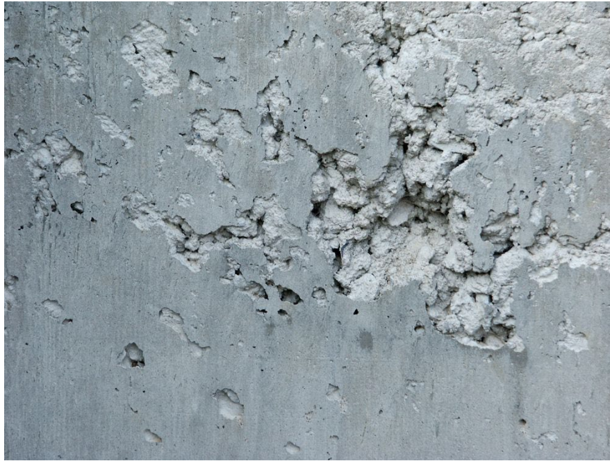
Figure 5-7 Bugholes and honeycombing at wall effected zone
