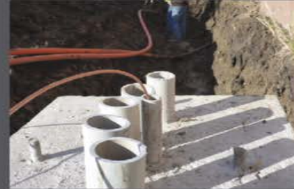
250,000 linear feet of conduit and fiber-optics
