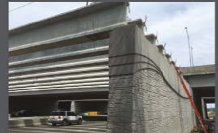
77 prestressed-precast concrete beams
