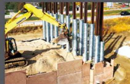
384,670 linear feet of retaining wall
