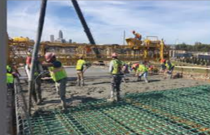
2,500,000 square feet of bridge deck
