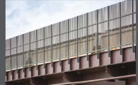
93,800 linear feet of permanent fencing
