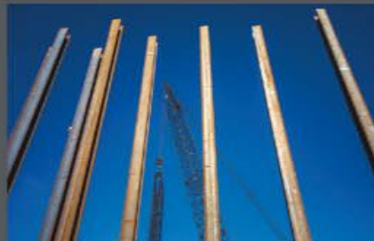
593,500 linear feet of steel pile to support bridges and other roadway structures
