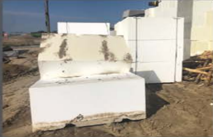
63,300 cubic yards of geofoam blocks
