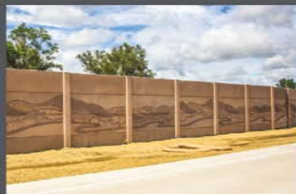
20,317 linear feet of noise wall
