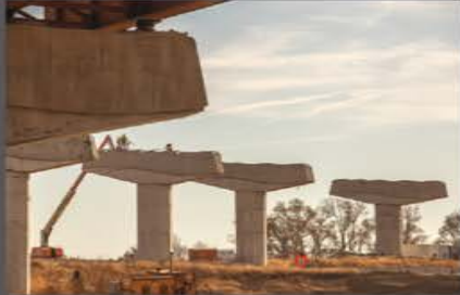
42,600 cubic yards of structural concrete
