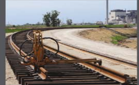
4 miles of new railroad track
