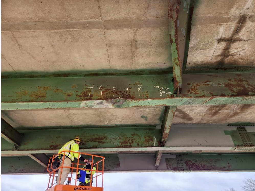
Beam 2, Span 2, Left (North) Side Bottom Flange Damage
