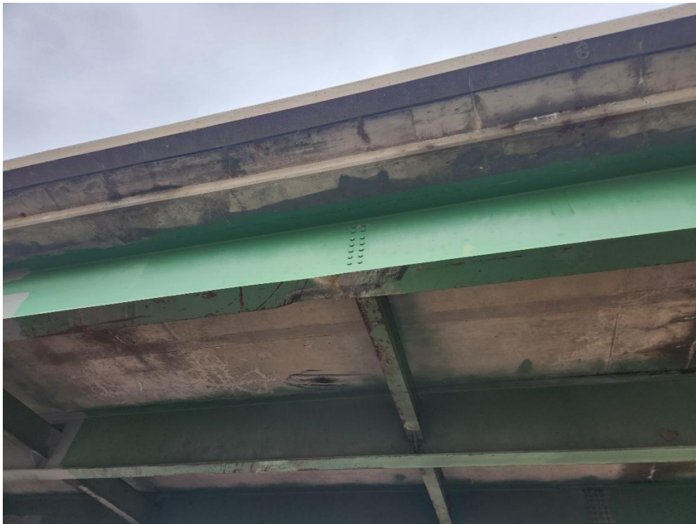
Beam 4, Span 2, Right (South) Side Bottom Flange Damage
