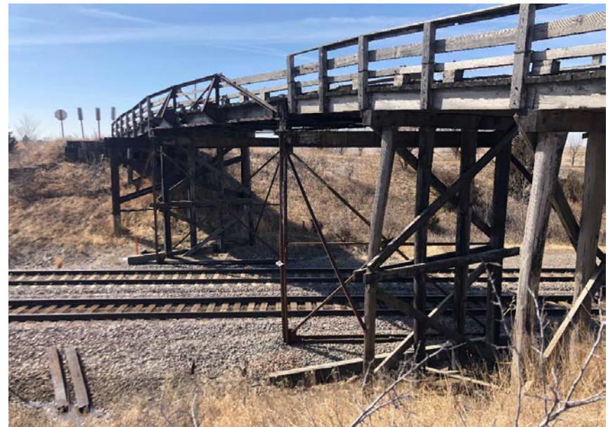
Montgomery County Wagon Bridge on L Ave near Red Oak, Iowa
