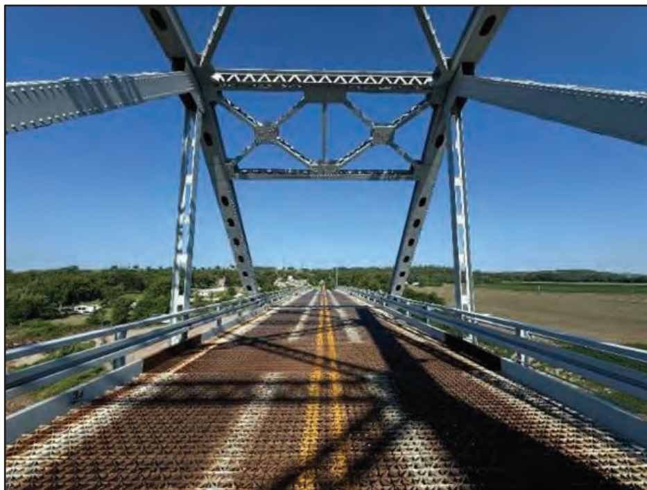
Figure 1-5: Decatur Bridge Looking West Towards Decatur, NE Along the Bridge Centerline
