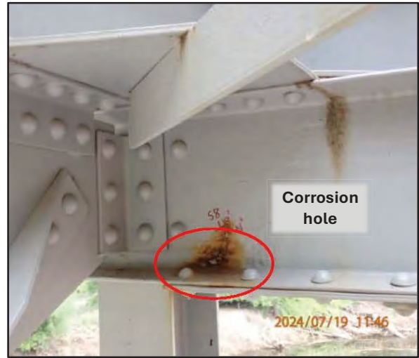
Figure 1-8: Examples of Structural Deficiencies Identified During 2024 Inspection
