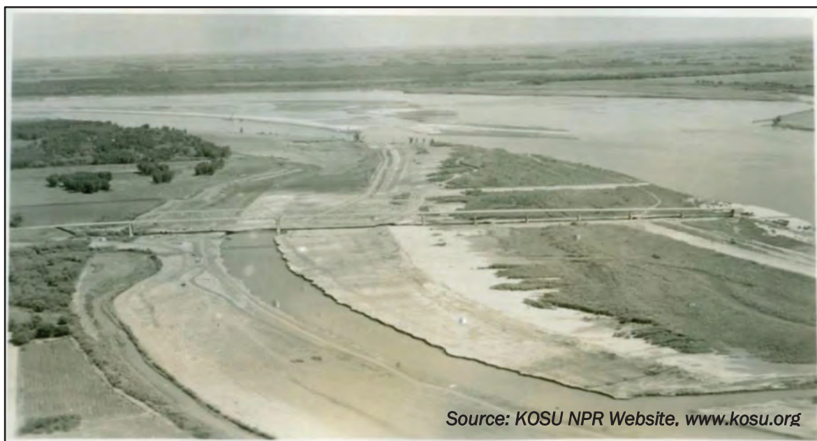
Figure 1-2: USACE Realignment of the Missouri River under the Decatur Bridge, 1955 (looking north)
