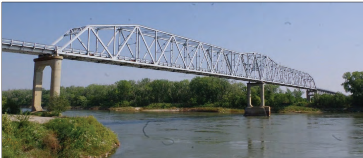
Figure 1-3: Decatur Bridge (S051 03644)
