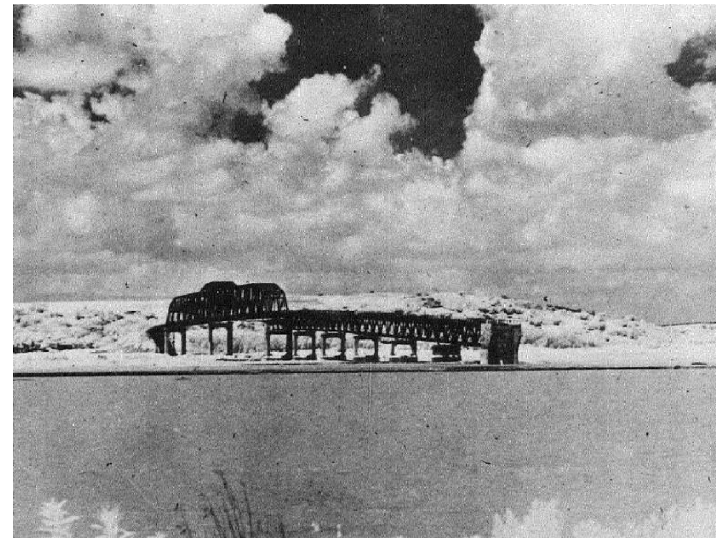
Photo: A “dry-land” bridge was built on the Nebraska side of the Missouri River in 1951 and the flow of the stream channeled under it in 1956. (Courtesy of the Omaha World-Herald and the Hudleson Studio, Onawa Iowa.)
