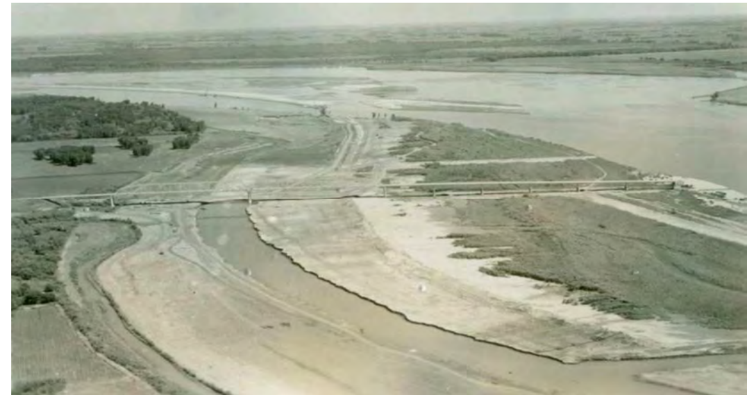
Photo: Partially completed bridge & USACE excavation, 1955.
