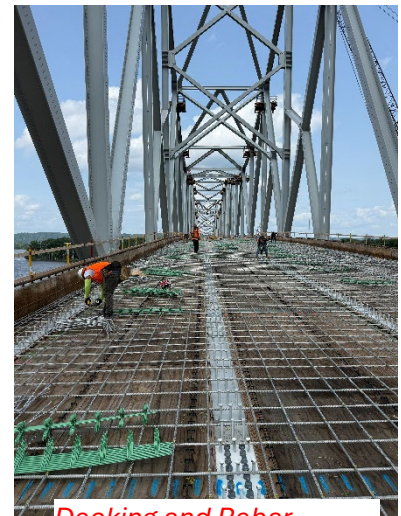
Decking and Rebar
