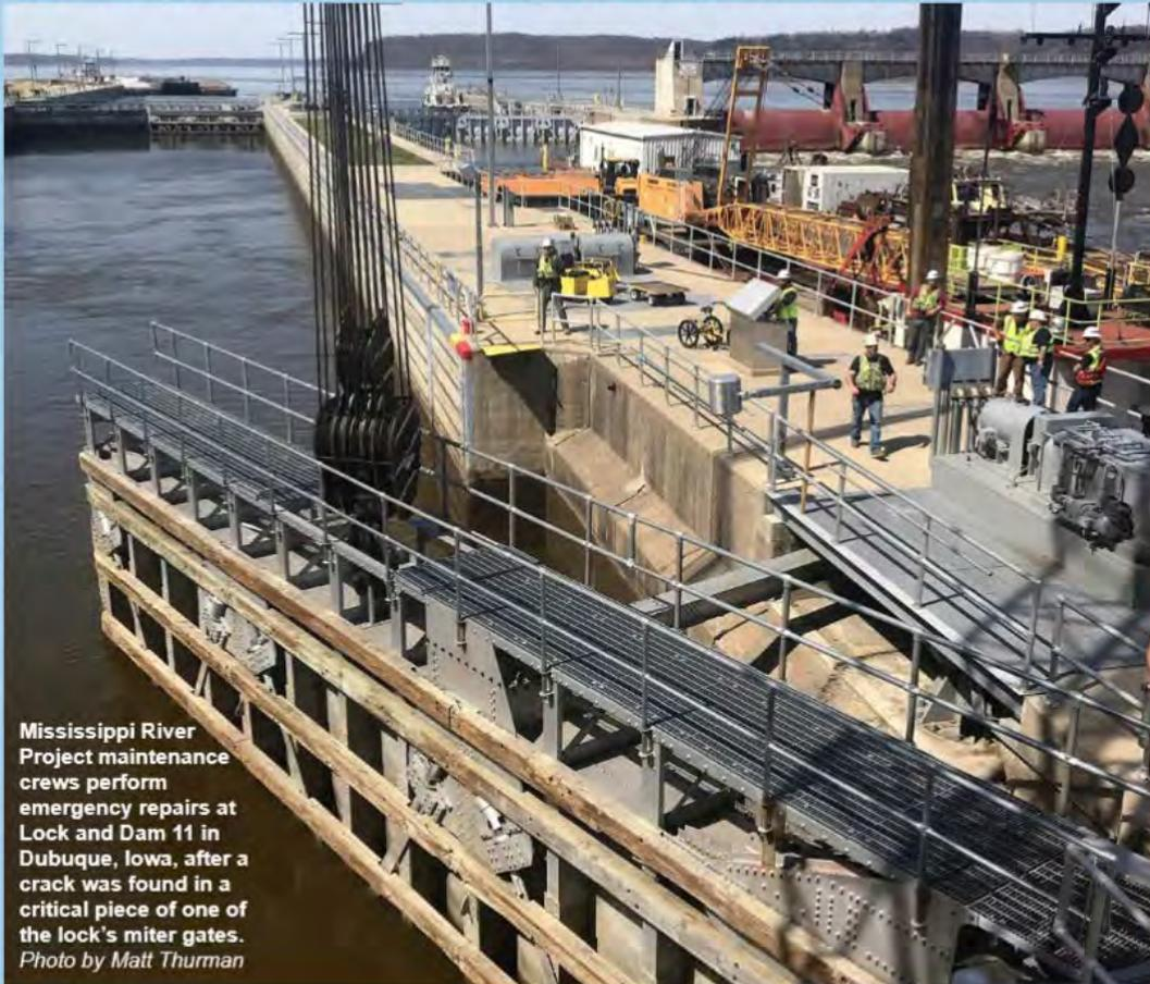
Mississippi River Project maintenance crews perform emergency repairs at Lock and Dam 11 in Dubuque, Iowa, after a crack was found in a critical piece of one of the lock's miter gates. Photo by Matt Thurman
