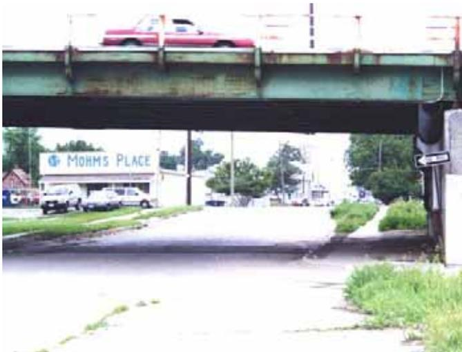
**Photo 3. Bridge lacks established vertical clearance over 10<sup>th</sup> Street**
