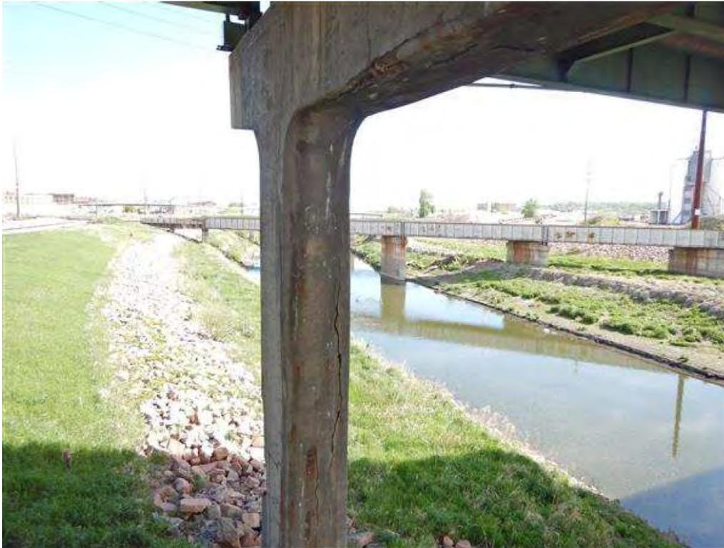
Following the 1999 and 2001 inspections, major repairs were completed, including a viaduct rehabilitation project in 2005, a new bridge deck overlay in 2008, deck joint repairs in 2013, and pier repairs in 2018. Epoxy injection, which has an expected lifespan of approximately 5 years, was completed in early 2023. However, these repairs provide only a temporary solution, and the lifespan of the intermittent repairs will expire relatively soon.
