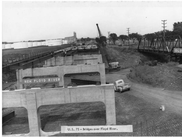
**Plate 7.** Construction of U.S. Highway 75 Bridge over Floyd River, 1956
