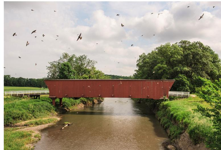
The Hogback Bridge was also built by Harvey P. Jones and George K. Foster using the Town lattice truss with queenpost overlay. It was the last covered bridge built in Madison County. The Hogback spans 98 feet over the North River, four miles northwest of Winterset. While most of the covered bridges were named for nearby landowners, the Hogback was named for the Hogback Ridge at the west end of the valley (its convex curve resembling the curve of a hog’s back).
