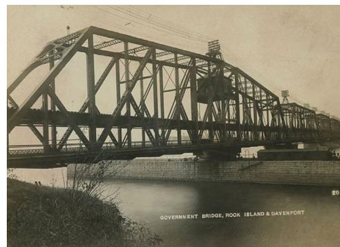
The bridge was built by utilizing timber and iron, which rested on granite piers. The draw-span allowed an opening of 120 feet (37 m) on both sides to let steamboats pass through. The lower deck of the bridge, which was 35 feet (11 m) above water, was used for wagons while the upper
