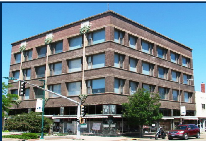
Van Allen Building, Clinton
