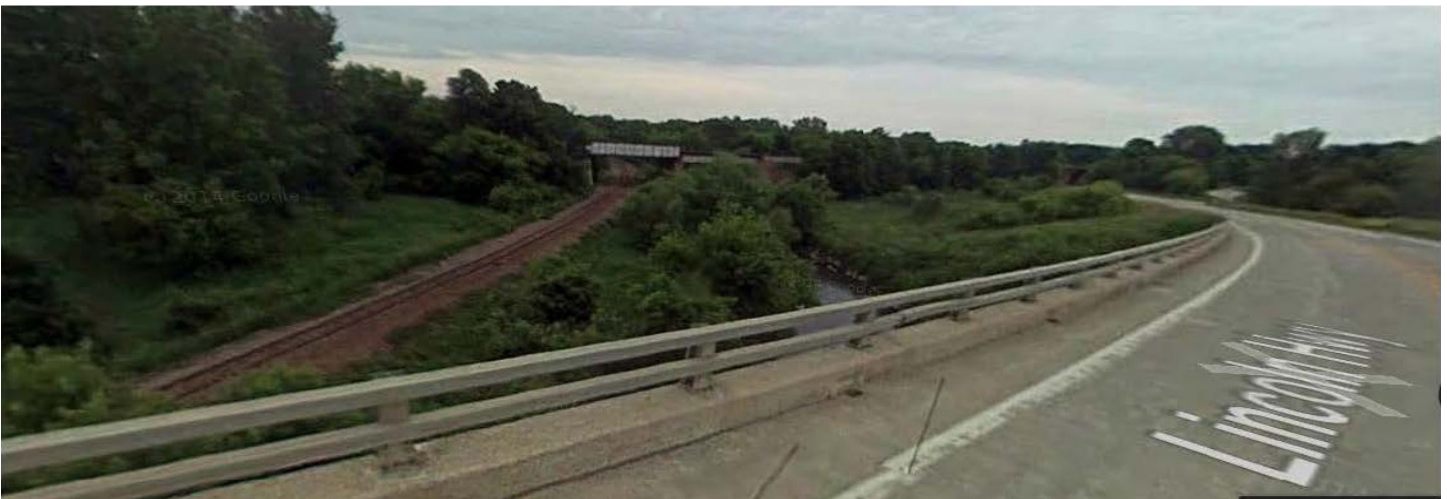
Overpass, looking east
