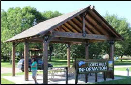
Information Pavilion containing interpretive wayside panels in Akron.
