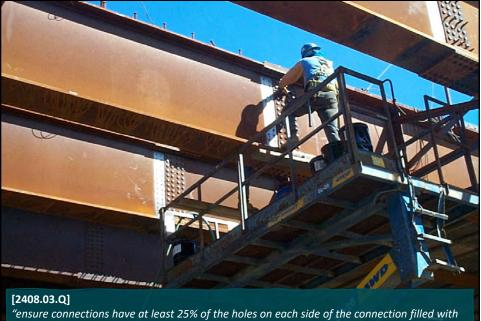
"ensure connections have at least 25% of the holes on each side of the connection filled with drift pins, and another 25% of the holes on each side filled with bolts drawn up snugly before the temporary support is removed..."
