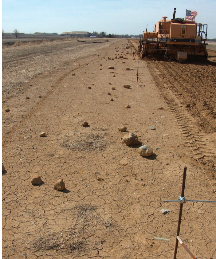
Figure 6-4: Rocks that required removal prior to paving
