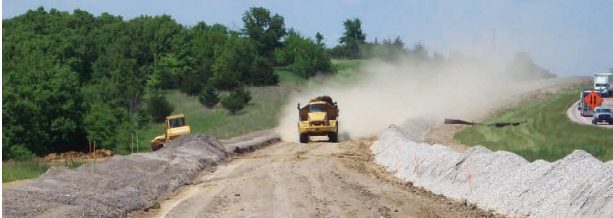
Figure 6-19: Haul roads or the project site may require application of water for dust control.
