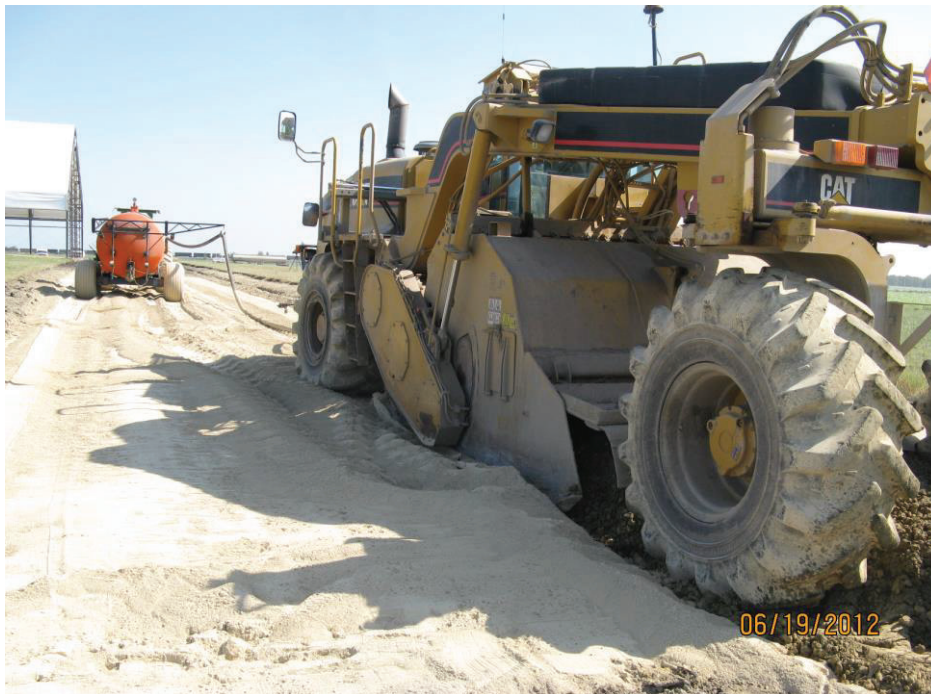
Figure 10-2: Pulverizer mixing fly-ash with subgrade soil.
