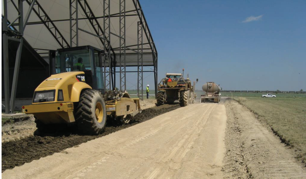
Figure 10-3: Compaction following behind pulverizer.
