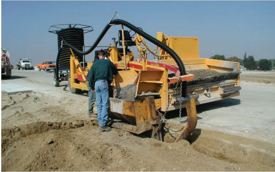
Figure 9-5: Installation of longitudinal subdrain
