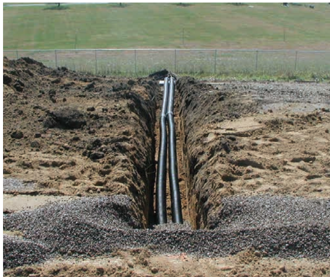
Figure 9-6: Longitudinal subdrain outlets
