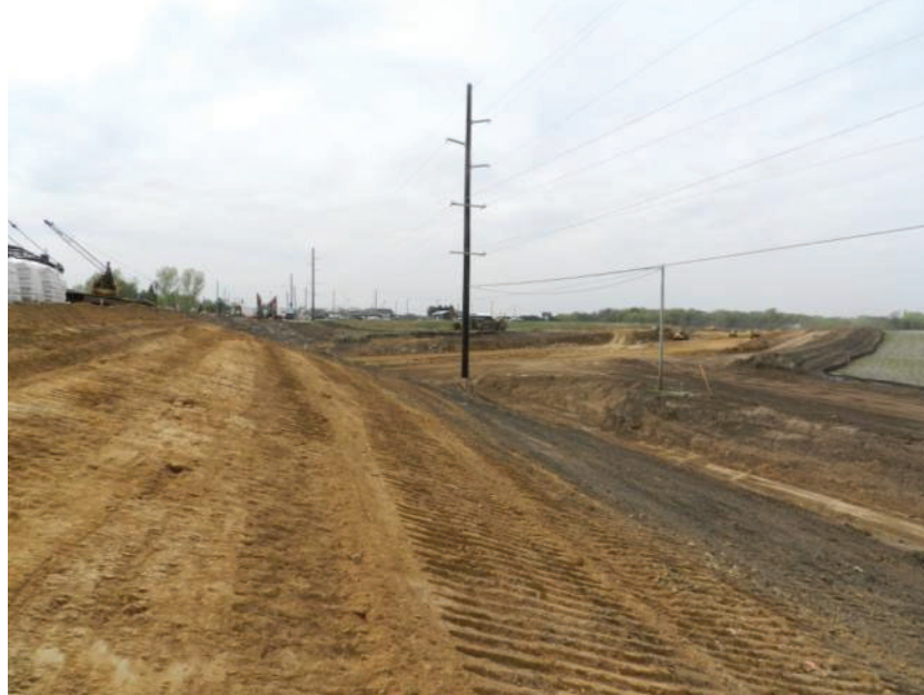
Figure 5-1: Grading may occur around existing utilities.
