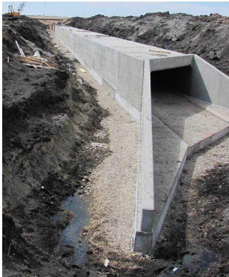
Figure 6-16: Contractor should not place backfill at box culverts until at least 14 days after concrete has been placed.
