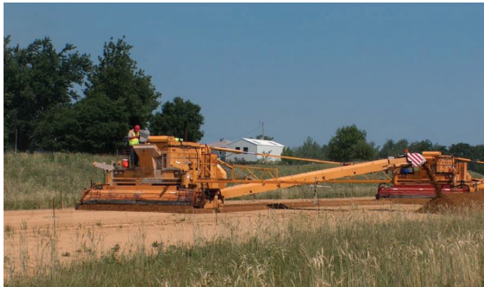
Figure 12-3: Subgrade trimming operations
