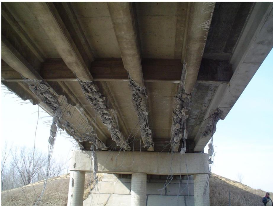
**Figure 2.9.3.2-7. Multiple Prestressed Beams with Severe Damage**
