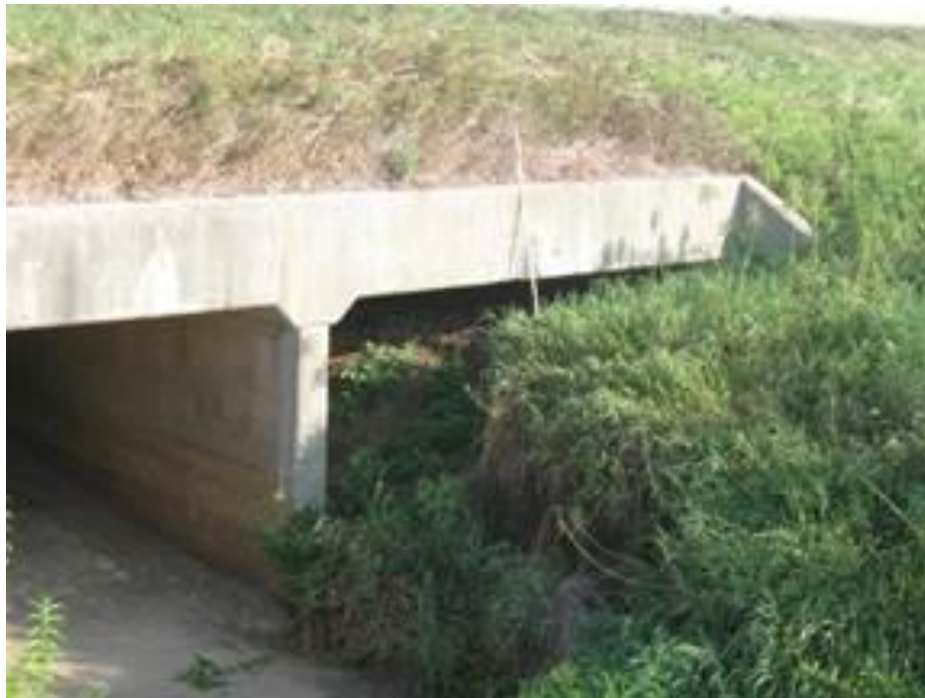
Figure 2.4.5-1 Silt Accumulation
