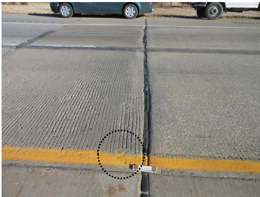
Figure 2.4.1-3 EF Joint Pavement Marking
