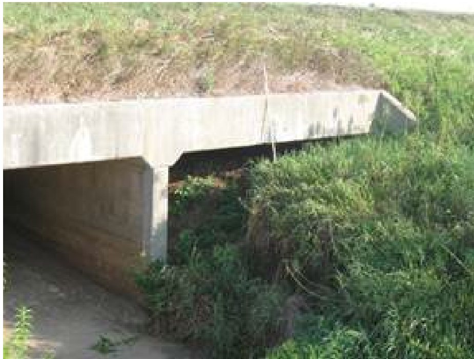
Figure 2.4.5-1 Silt Accumulation
