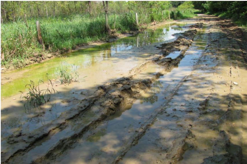
**Deposits of silt on an access drive made this area impassible. Cost to repair included removing deposited silt and installing new rock.**
