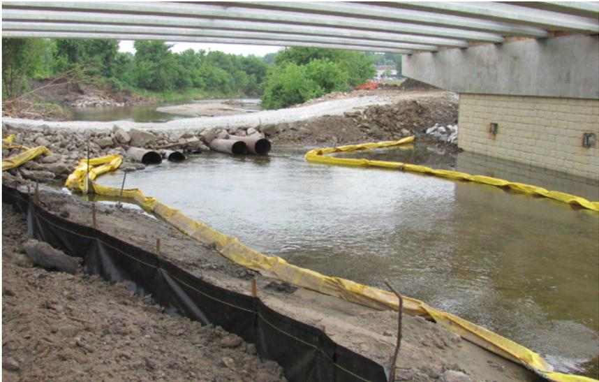
**A temporary stream crossing was constructed by the contractor to allow for access to both sides of the creek. When a temporary stream crossing is used, it should be completed according to EW-401.**
