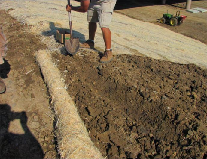
**It is important to ensure that the contractor installs the slope protection properly – this includes using anchor slots at the top of the slope protection to ensure flows do not travel underneath.**
