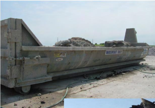
**A concrete washout may look like these photos or be as simple as a hole dug to contain the washout as long as it does not adversely affect a water of the state.**
