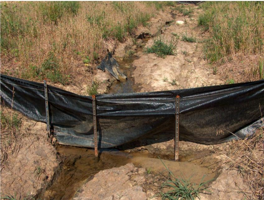
**This ditch check has been undermined and should be removed. This area may benefit from different controls - the ditch bottom should be seeded and mulched or possibly matted.**
