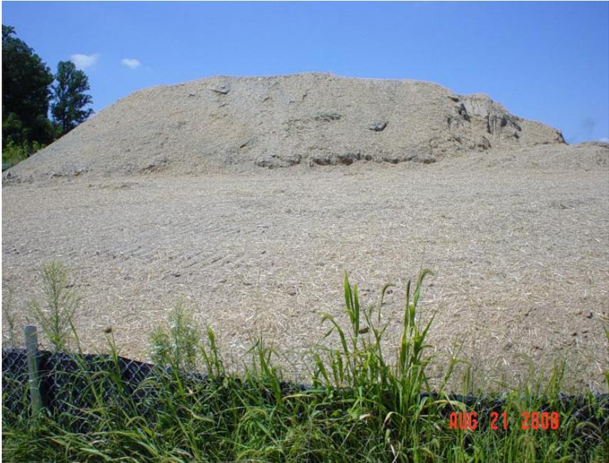
**Stockpiles should be stabilized if they will not be used within 14 days. Silt fence may also be required around stockpiles to protect the surrounding area.**
