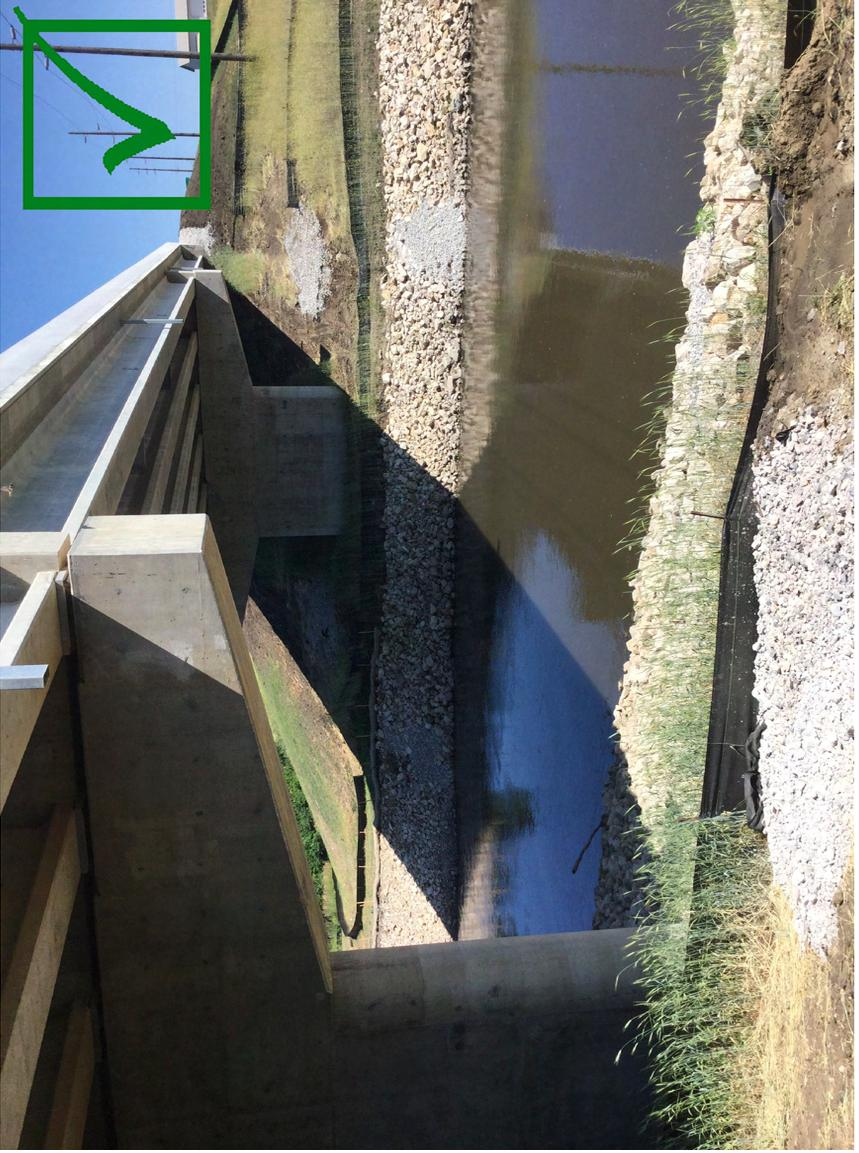
This photo shows silt fence that has either been blown-out or run over by equipment. If this occurs, the silt fence should be repaired immediately because it is the last line of defense to prevent silt from entering the creek. It would also be a good idea to have two lines of controls along a waterbody.
