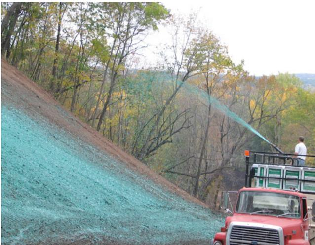
**Hydraulic seeding - Typically, inoculant, seed, and fertilizer are to be applied in a single operation. Hydraulic mulch is then applied as a separate operation.**
