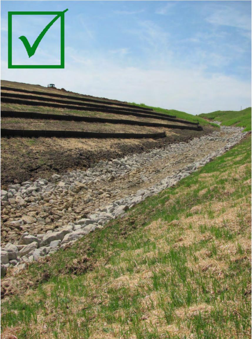
Multiple rows of silt fence installed along the contour of a slope. Due to the ditch grades, a rock ditch was installed to prevent erosion in the ditch. The backslope was also seeded prior to the road embankment being completed.
