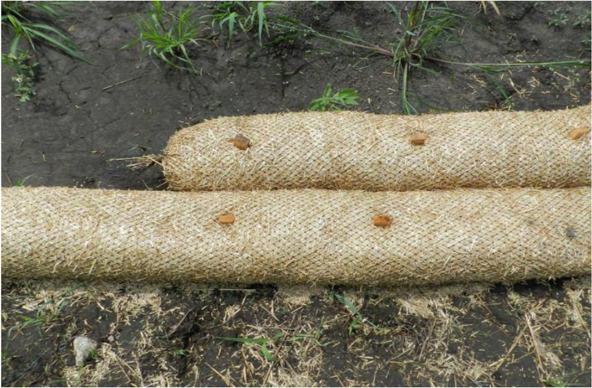
**Ditch check showing wood stakes at correct spacing and controls overlapped.**
