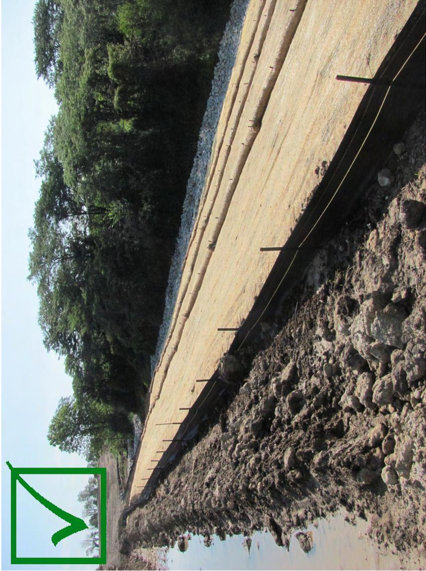
A stream diversion channel was constructed so that the contractor could install a new culvert. This photo shows no controls along the top of the channel (on the left) and spoil piles without silt fence or logs and no stabilization (on the right side of the channel).
