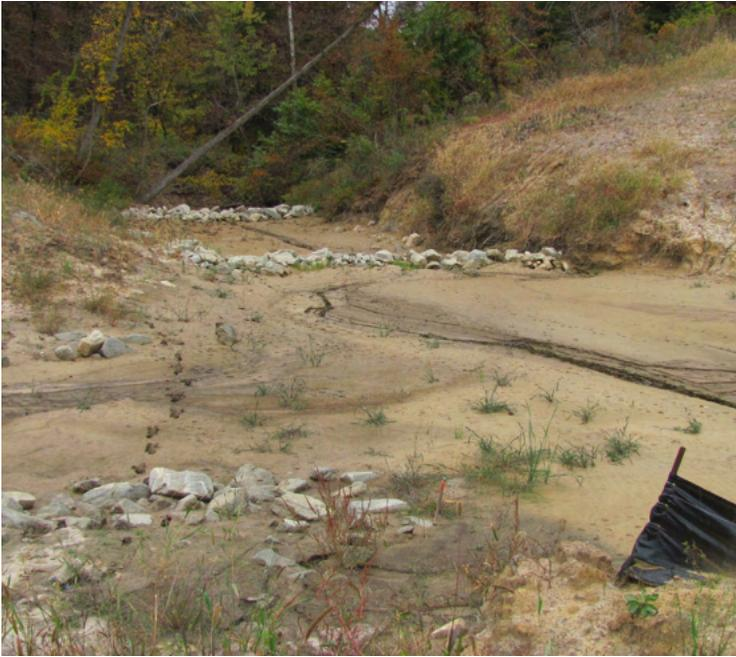
**This silt basin's capacity has been reduced by more than 50% and requires clean-out.**
