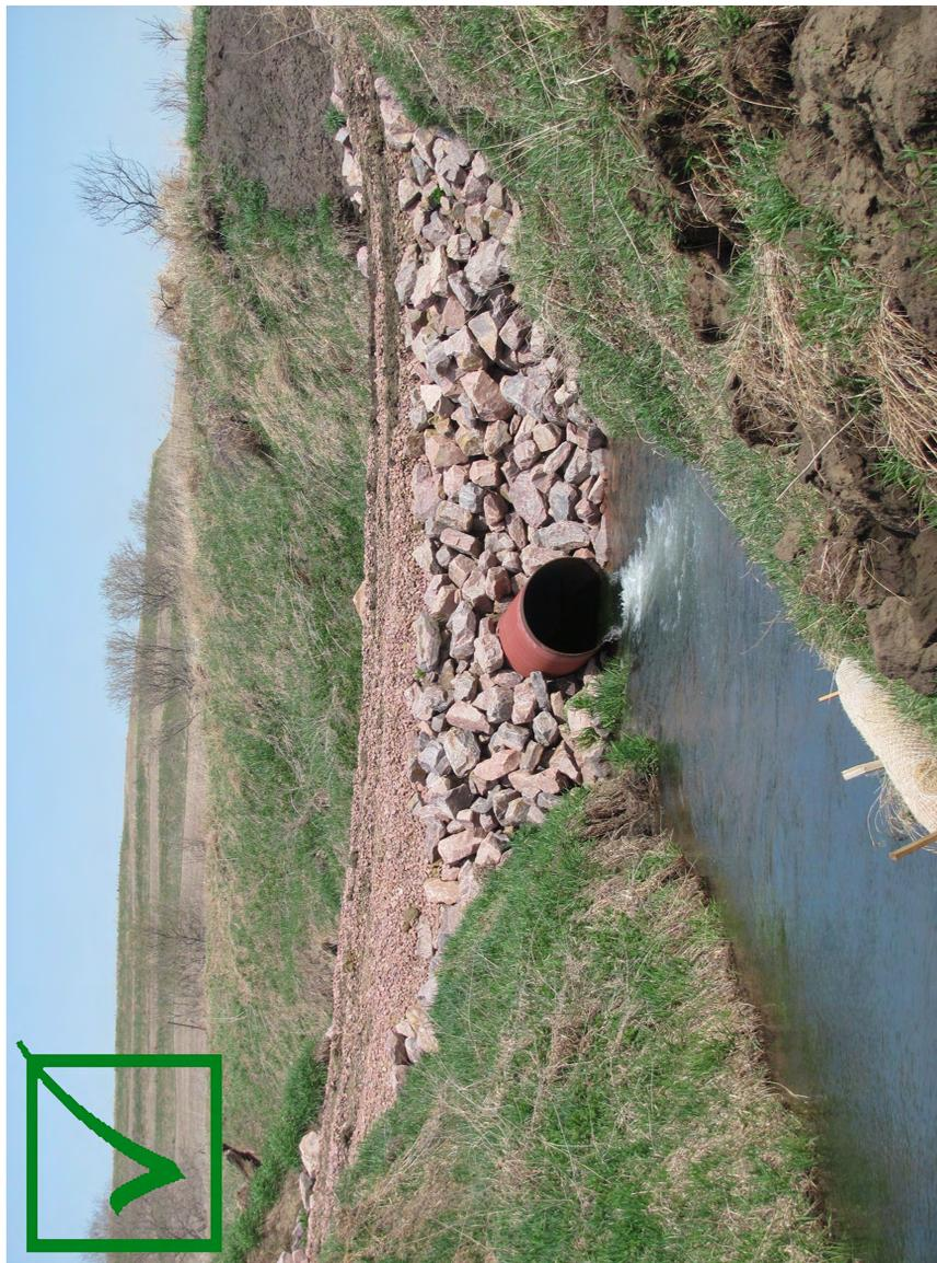
This photo shows a very poor example of a temporary stream crossing on a culvert extension project. Only clean fill per EW-401 should be used in the water.
