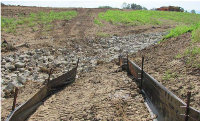
**Silt Fence is a type of structural control.**
