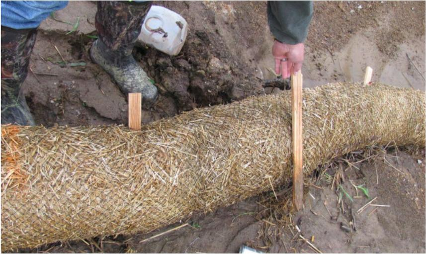
**EC-204 requires wood stakes be driven into the ground a minimum of 12 inches. This photo shows stakes incorrectly driven into the ground several inches.**
