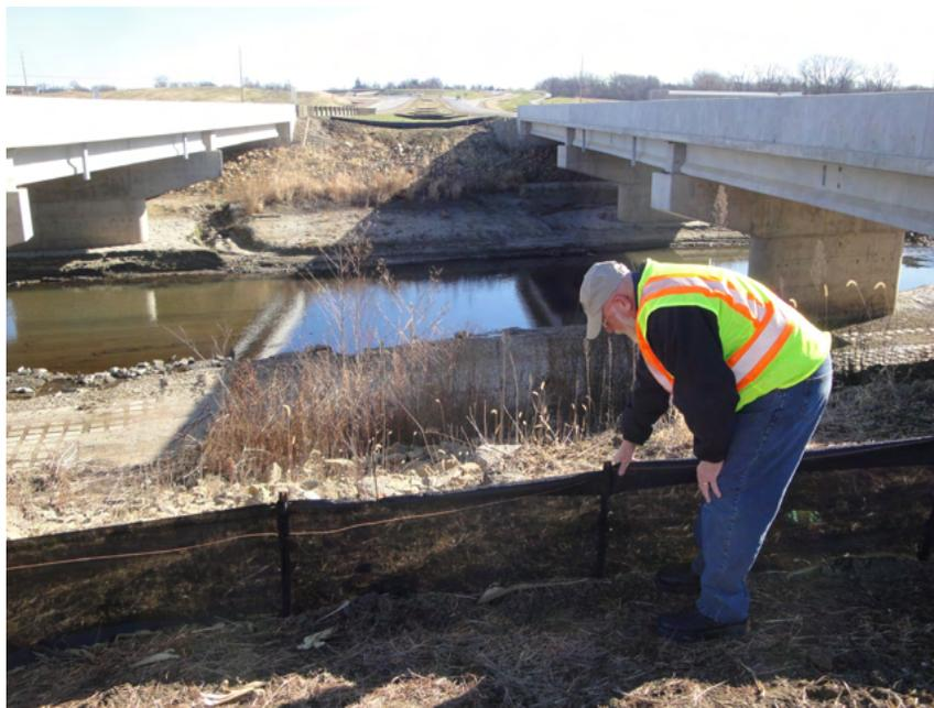
**Give the silt fence fabric a good tug to ensure it's properly installed. When properly installed, silt fence fabric should be tight between the posts.**
