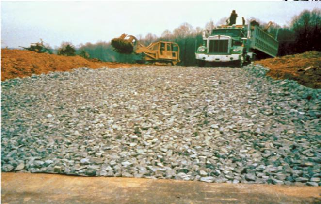
**A stabilized construction entrance is designed to minimize tracking of sediment from the site by vehicles and equipment.**
