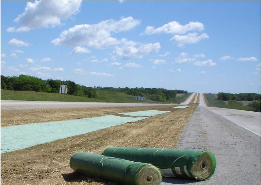
**Wood excelsior and coconut fiber mat is more durable to withstand the concentrated flow found in ditches.**
