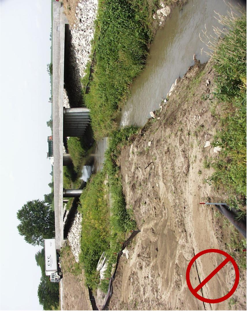
Water drained off the top of the embankment and created rills in the foreslope. This is an example of how an area may appear stabilized but is still susceptible to erosion. These areas should be repaired and if possible, flows should be diverted to a stabilized area.
