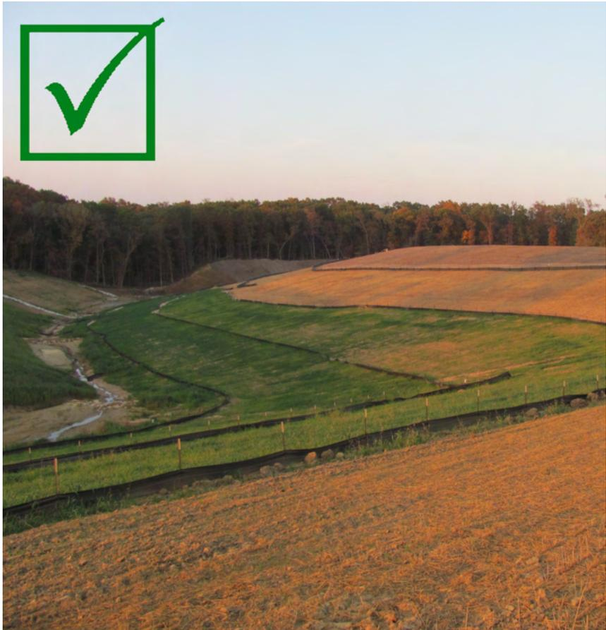
Embankment was stabilized in stages. Contractor did not wait until entire slope was completed before seeding and mulching. Silt fence was installed along contours (though it should have been broken up into smaller sections or installed with bumps - there is a maximum of 200 feet per section as shown in Standard Road Plan EC-201).
