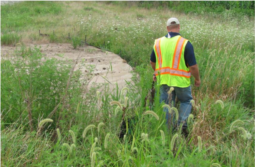
**Silt fence must be cleaned out or replaced when it becomes half full.**
