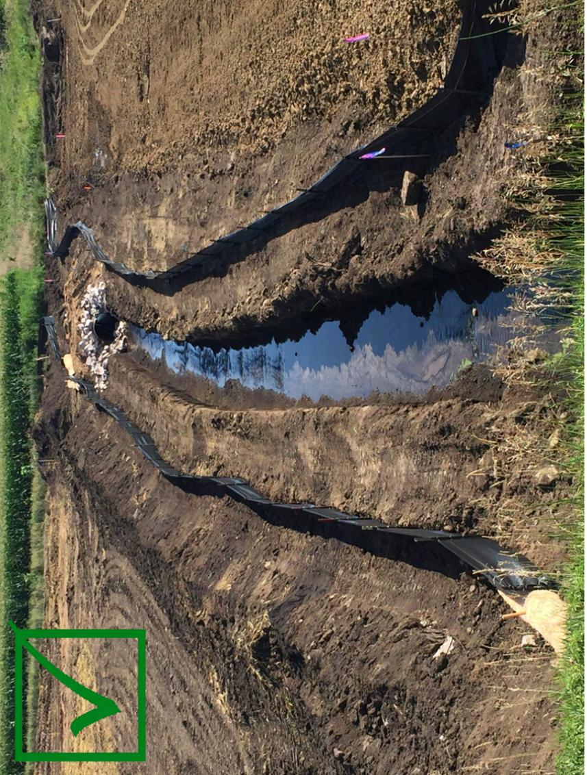
This is a disturbed area alongside a creek without any sediment or erosion controls. Perimeter controls should have been installed to prevent silt from entering the water body.
