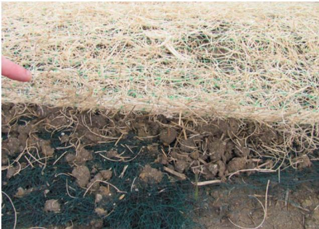
**This detail and photo show installation of TRM, which includes TRM, topsoil, and special ditch control.**
