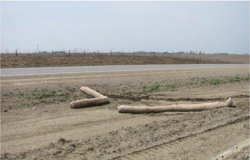
**Both logs used in this ditch check were not properly staked causing them to blow out.**
