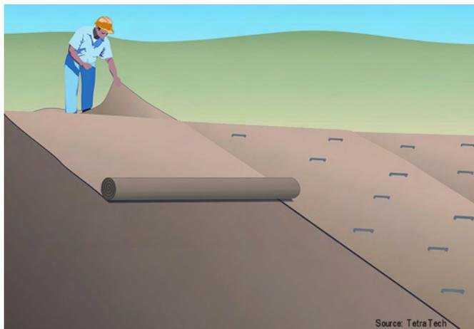
**Mat should be smooth and in contact with the soil surface. It should also be stapled in place.**
