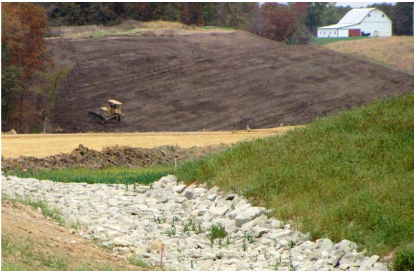
**Topsoil was stripped and stockpiled and is shown being respread in the background.**
