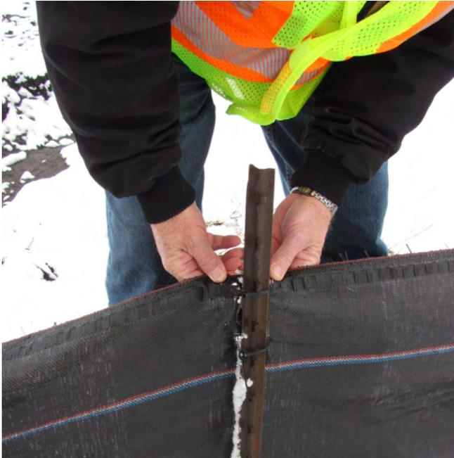
**This silt fence was incorrectly tied to the post with only two ties.**
