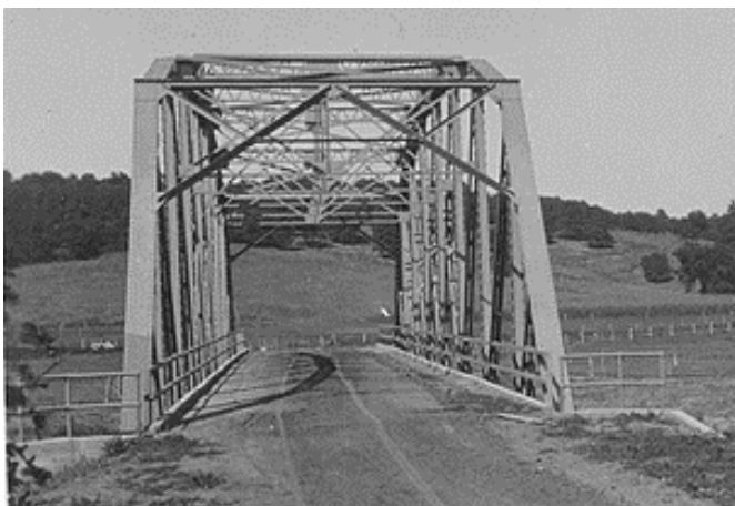
Steel Thru Truss
