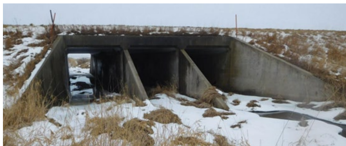
Concrete Box Culvert
