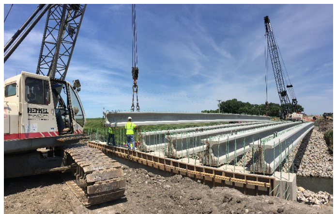
Prestressed Girder Construction
