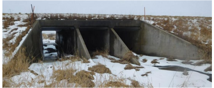
Concrete Box Culvert
