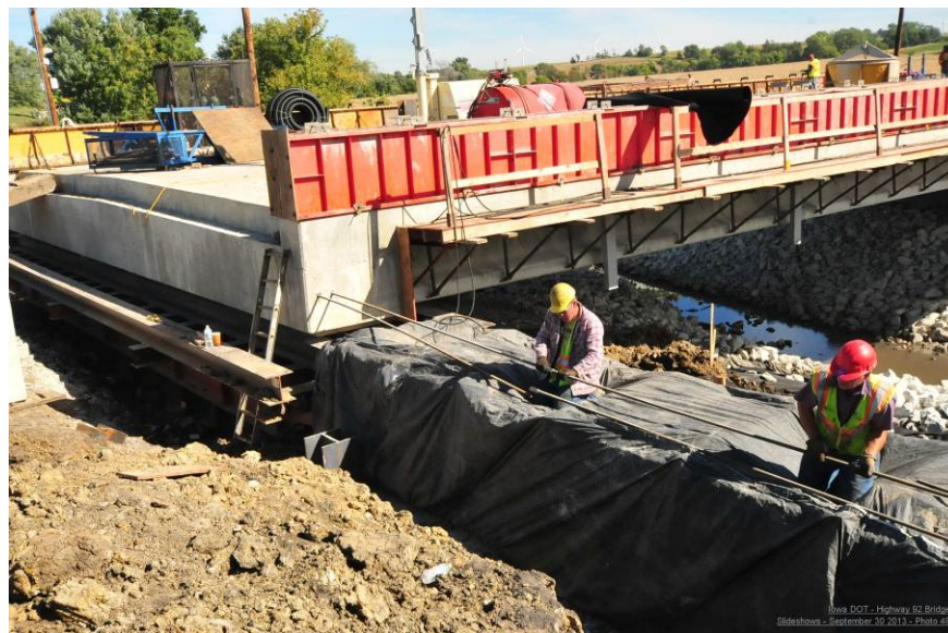
Figure 21 – Slide-in Bridge Construction Preparation
