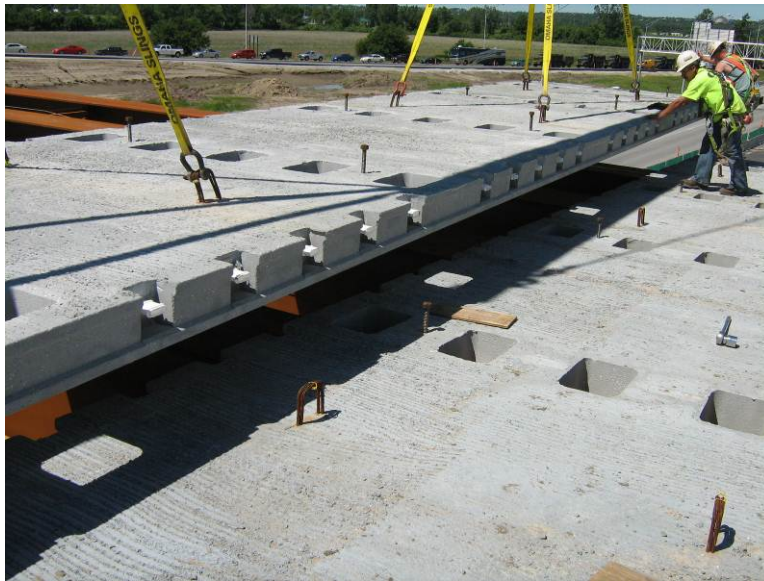
Figure 10 – Full-depth Precast Deck Panel Installation
