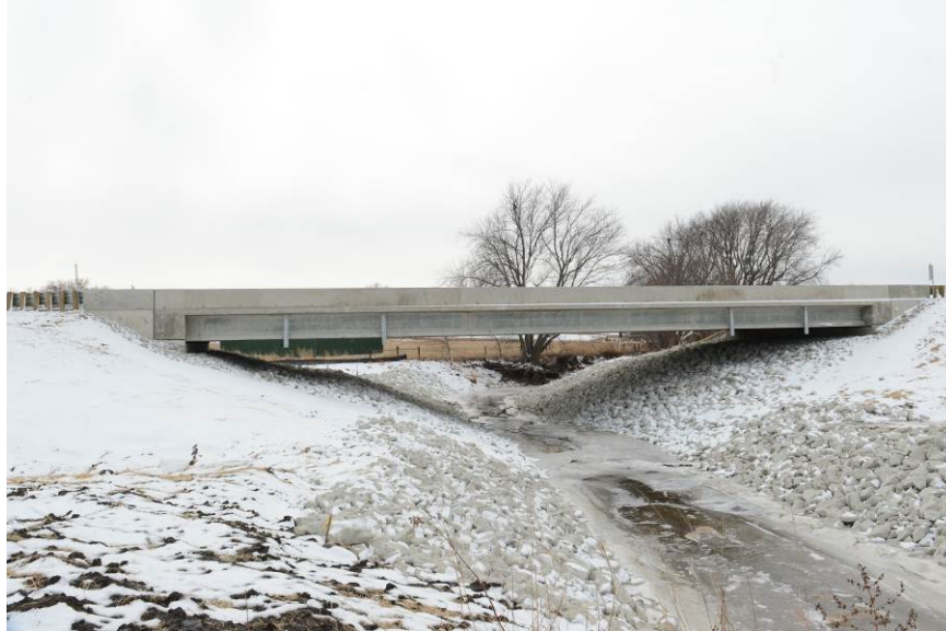
Figure 25 – Completed Massena Bridge
