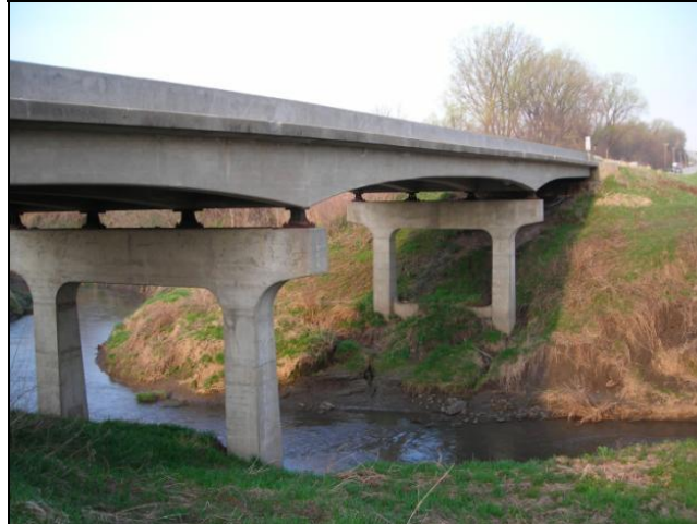
Figure 13 – Original US 6 over Keg Creek Bridge
