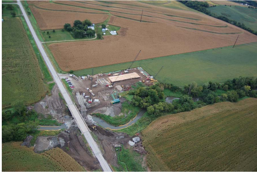
Figure 14 – Temporary Bridge Production Site.
