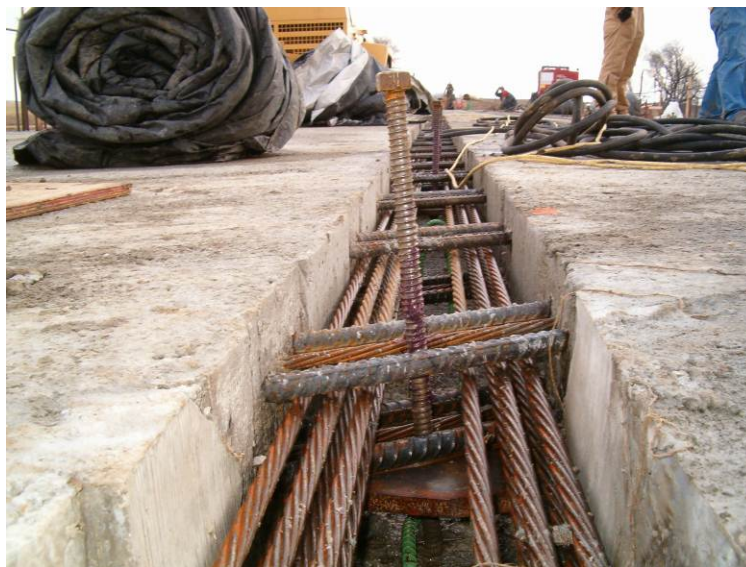
Figure 5 – Post-Tensioning Channel
