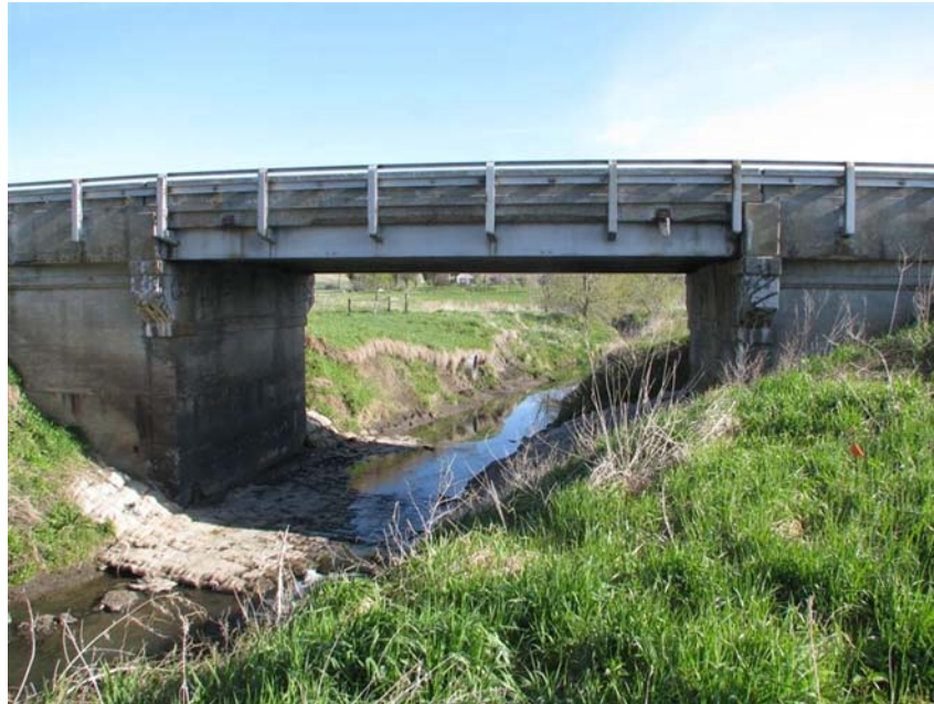
Figure 19 – Original IA 92 over Small Stream Bridge
