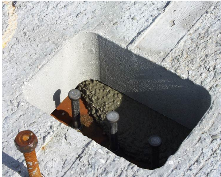
Figure 12 – Shear Stud Pocket
