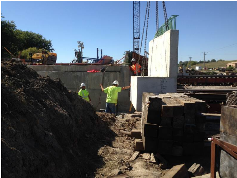
Figure 24 – Precast Wingwall Installation
