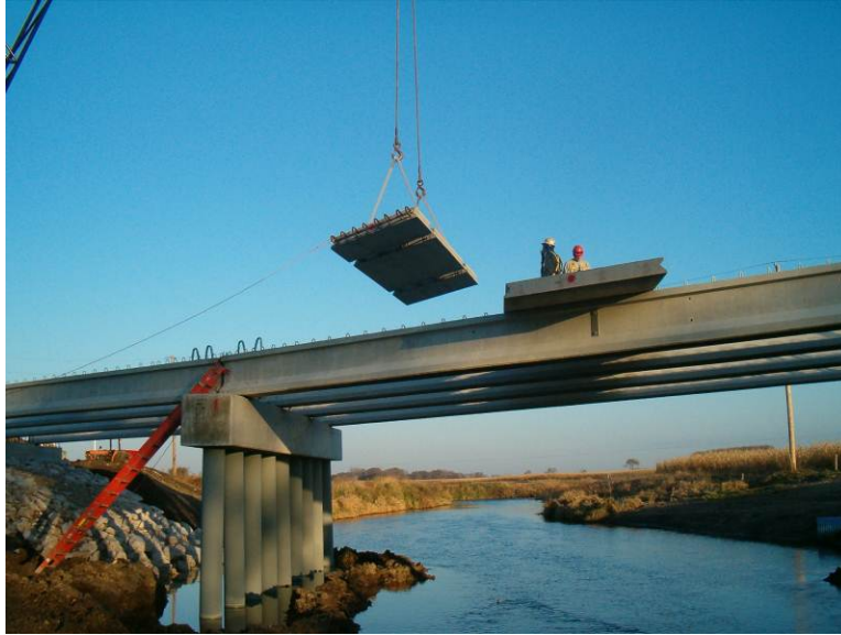
Figure 4 – Full-depth Precast Deck Panel Installation
