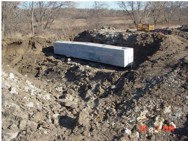
Figure 7 – Precast Abutment Footing
