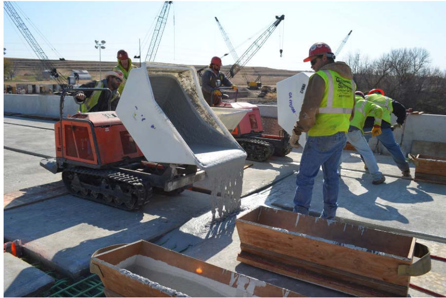
Figure 17 – Placement of UHPC
