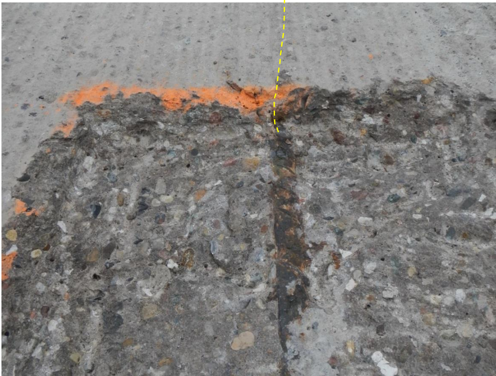
Figure E9. Corroding bar at crack (yellow line) in eastbound lanes.
