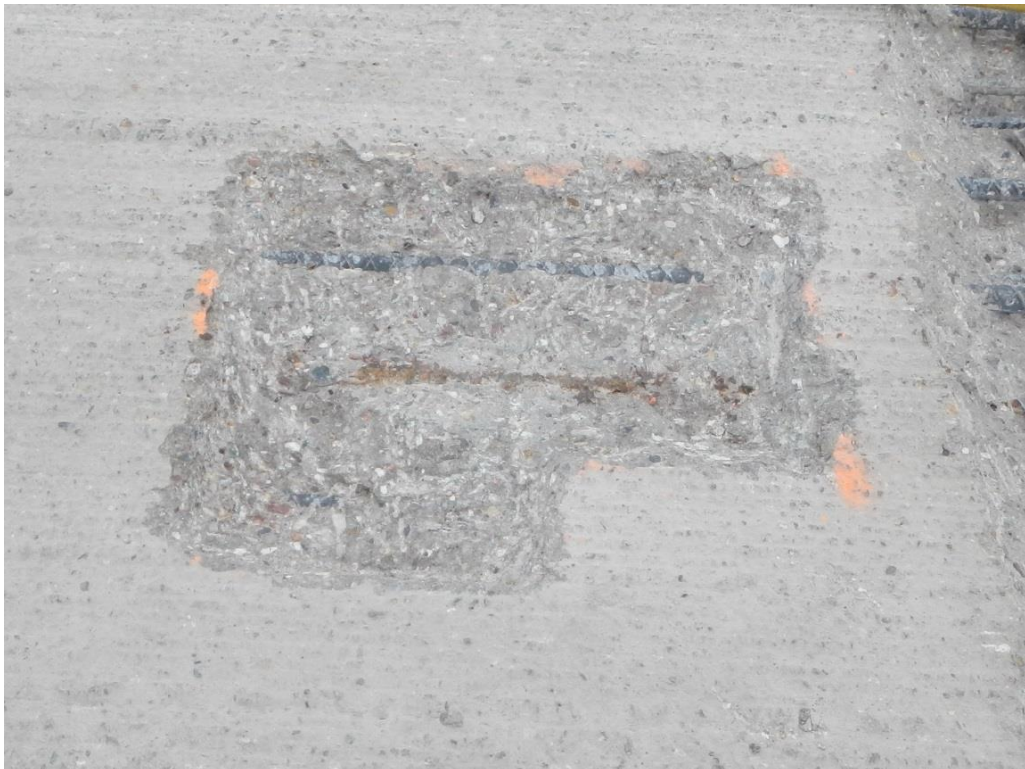
Figure E6. Close-up of repair location in IA92 deck, eastbound lanes.
