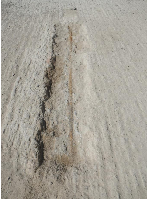
Figure E3. Typical repair location in IA 92 deck, westbound lanes
