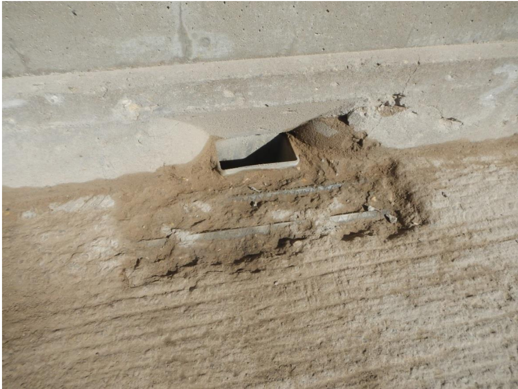
Figure E11. Concrete removal at scupper drain on westbound lane.
