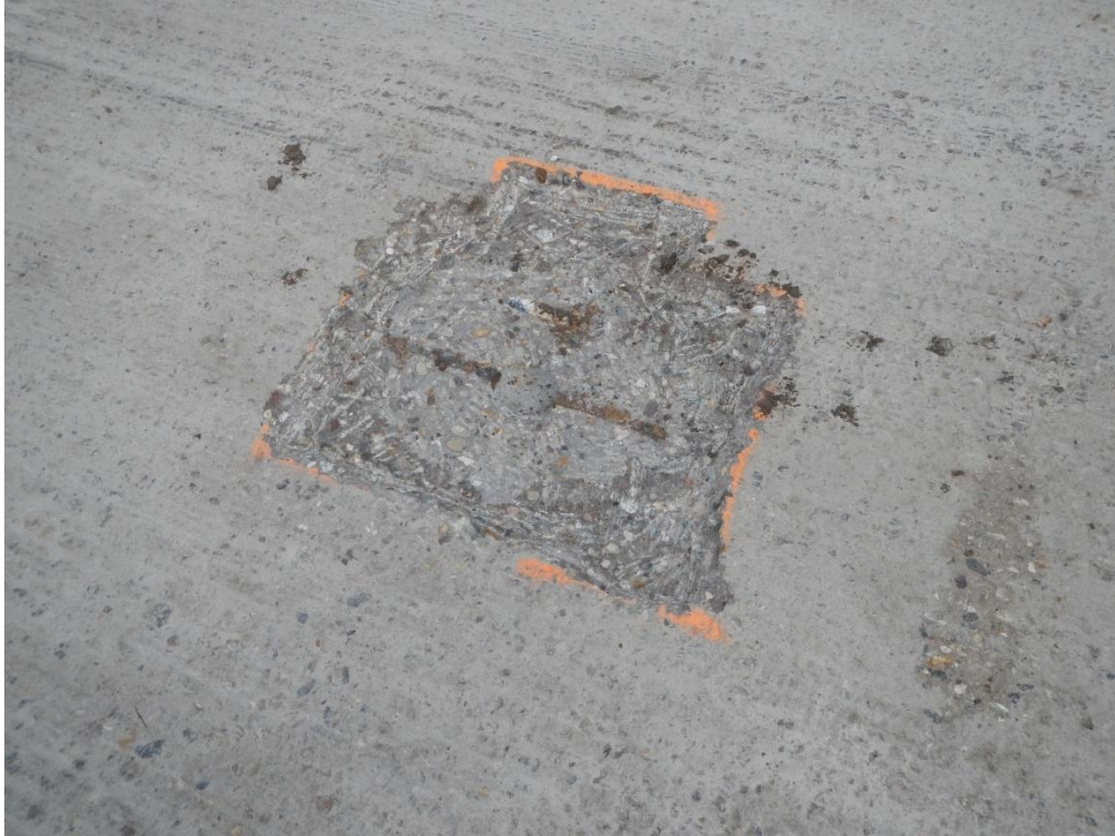
Figure E7. Typical repair location in IA 92 deck, eastbound lanes.
