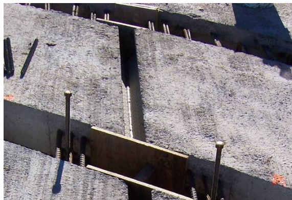
Figure 131. Transverse joint formwork, November 5
