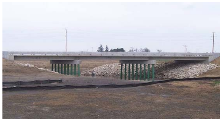
Figure 2. Completed replacement bridge on 120 th Street
