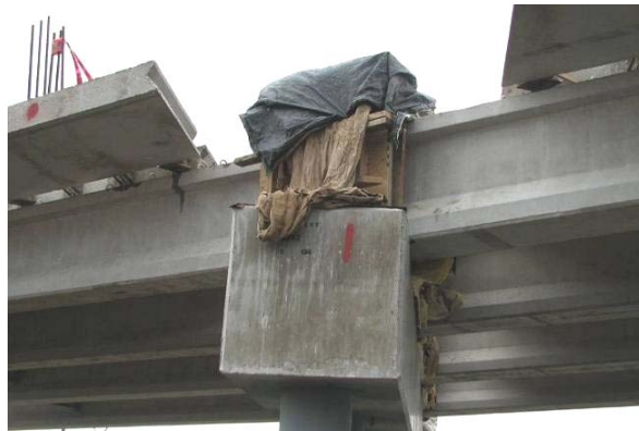
Figure 130. West pier diaphragm covered with burlap and plastic, November 4
