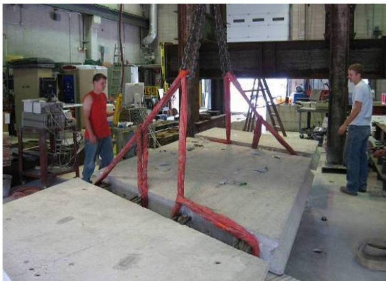
a) Photograph of lifting the deck panel with four straps
