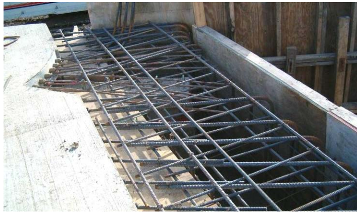
Figure 141. Reinforcement in the west abutment cap, November 29
