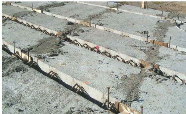
Figure 133. Several transverse joints before finishing, November 8
