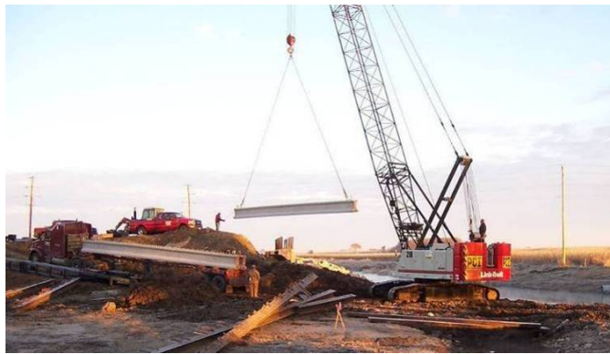
Figure 124. The first bridge girder being lifted into place, October 24
