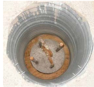
b) pipe pile in the pier cap
