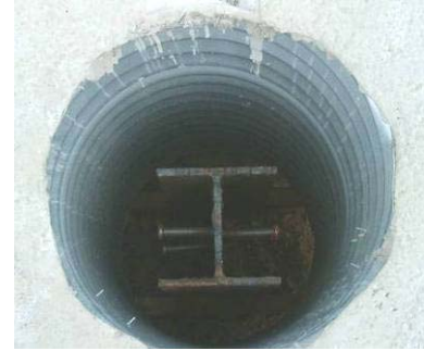
b) H-pile in the abutment
