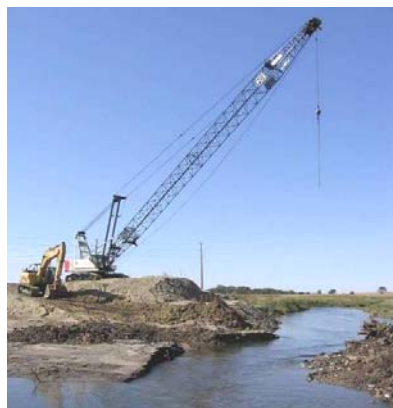
Figure 109. Damage to the west bank caused by the rain, September 20
