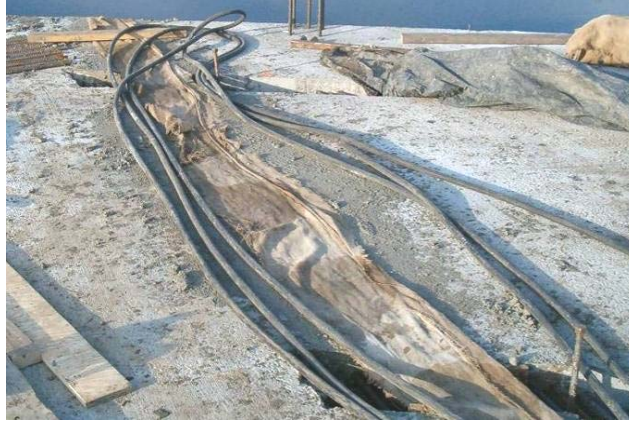
Figure 136. Burlap and heating coils on the west end panel joint, November 16
