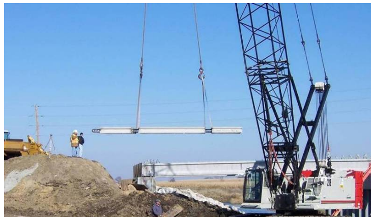
Figure 127. Deck panel being reset on the bridge girders, October 25
