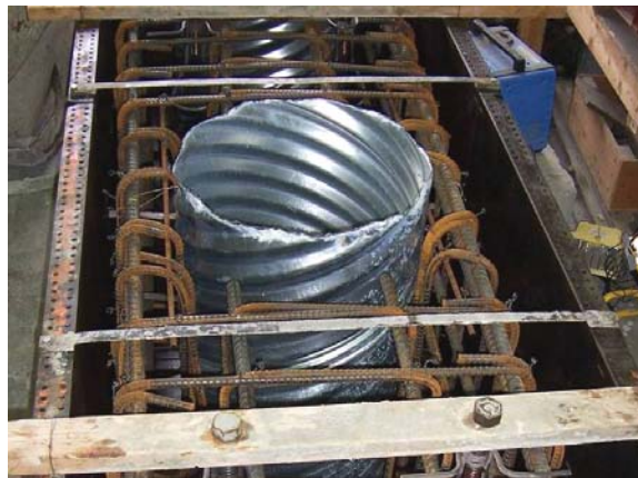
Figure 27. Pier cap reinforcement
