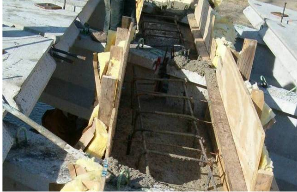
Figure 129. Pier diaphragm before concrete placement was complete, November 3
