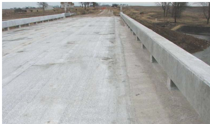
Figure 147. Bridge deck after the surface was ground, December 27
