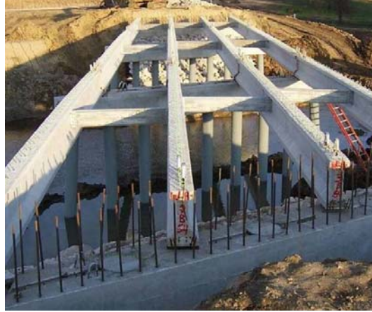
Figure 126. Erected bridge girders, October 24
