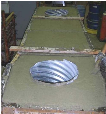
Figure 33. Abutment 6 after hand-finishing
