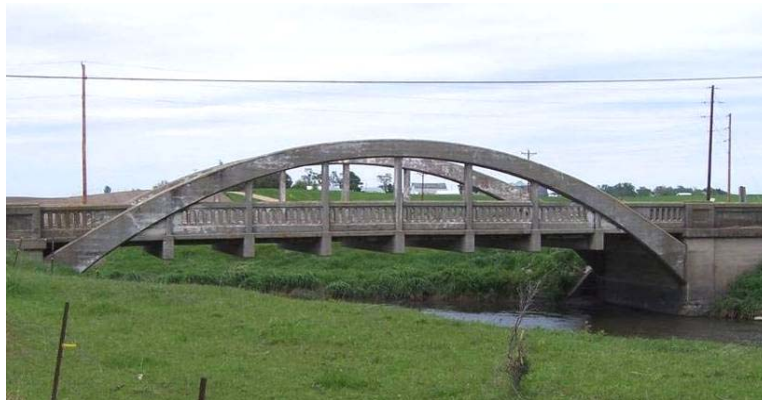
Figure 100. Previous bridge on 120 th Street, July 19
