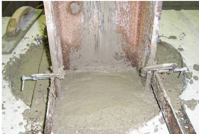
Figure 23. H-pile after being grouted in place
