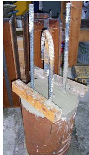
b) Pipe pile after placing concrete
