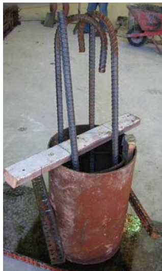
a) Pipe pile before placing concrete
