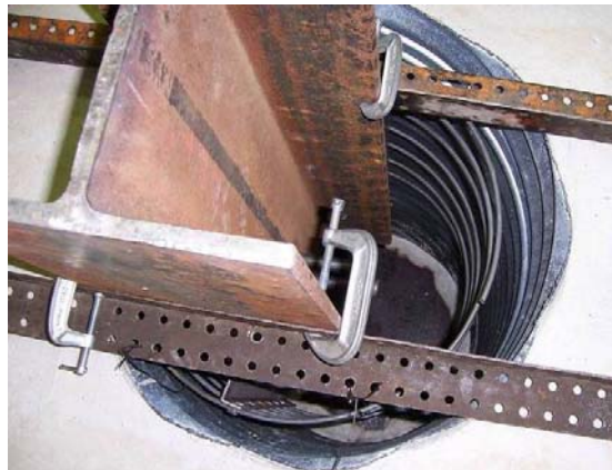
Figure 21. H-pile in place before placing grout
