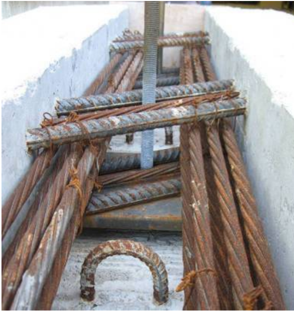
b) Steel in channel
