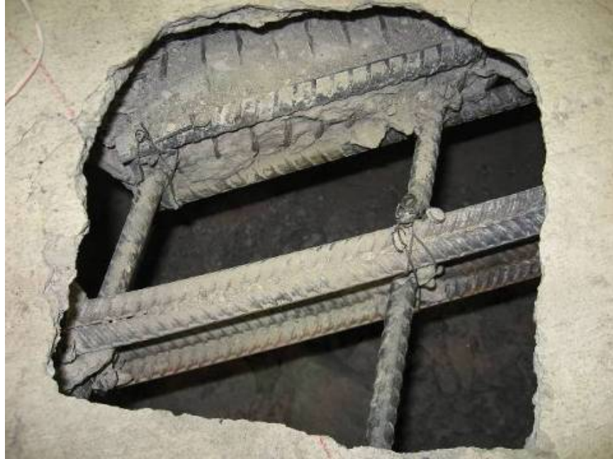
b) Top view after concrete removal
