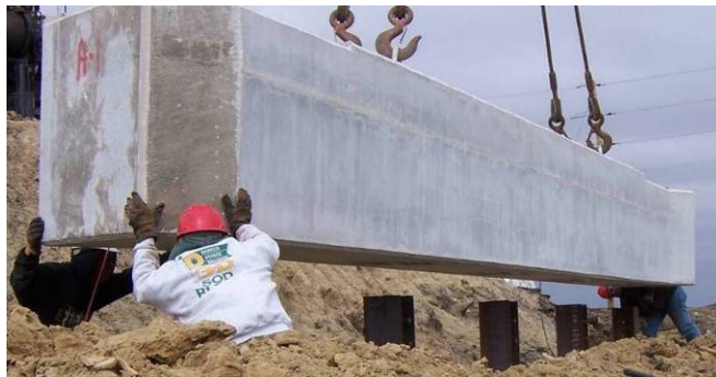
Figure 114. West abutment being lowered in place, October 4
