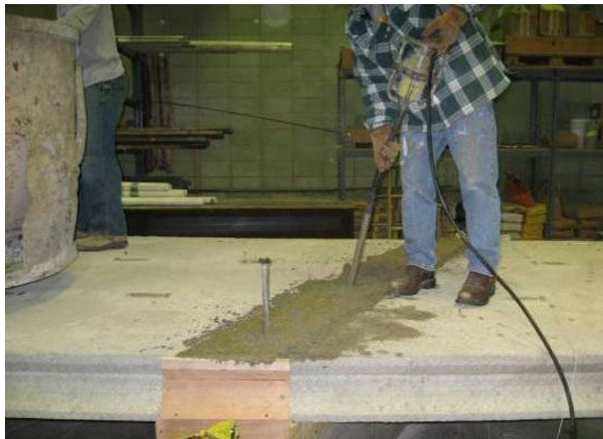
b) Placement of concrete in channel
