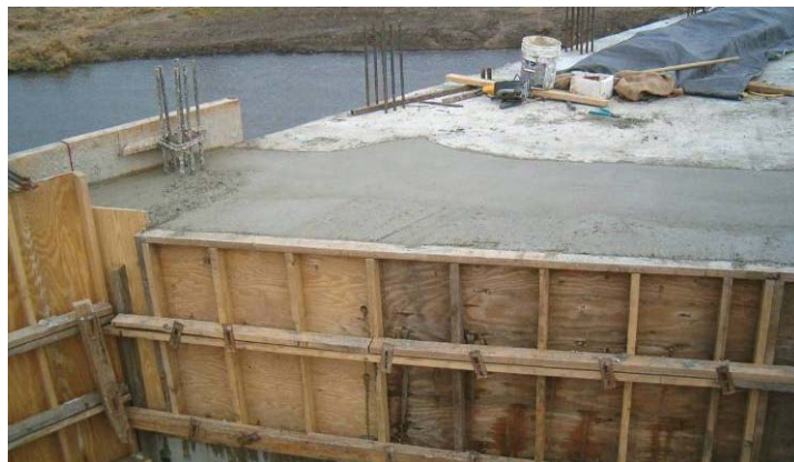
Figure 142. West abutment and wingwall, placed and finished, November 29
