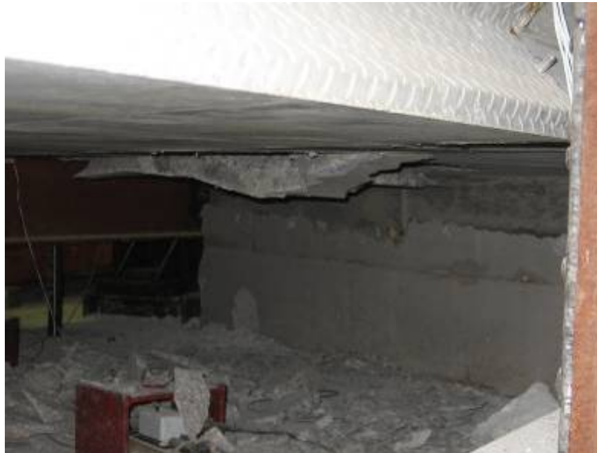
c) Underside of the deck panel
