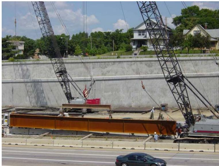
**Figure 3.18. HPS girder being unloaded following delivery**
