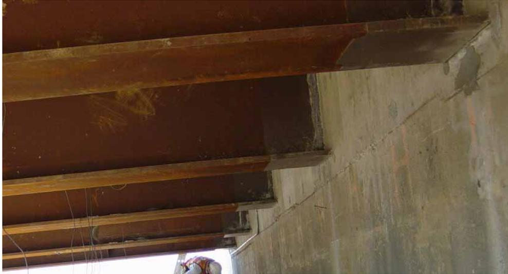
**Figure 3.2. Typical girders and the north integral abutment**
