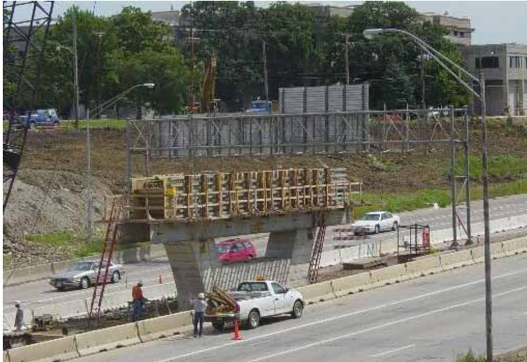
**Figure 3.16. Formwork for the center pier cap being constructed**
