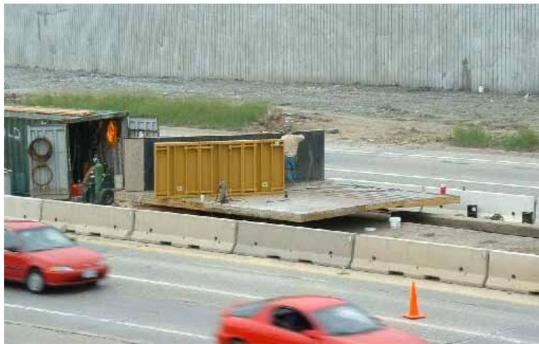
**Figure 3.13. Formwork for the center pier during assembly**
