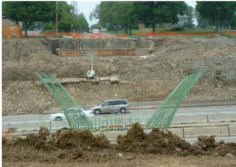
**Figure 3.11. Reinforcing steel for the center pier**
