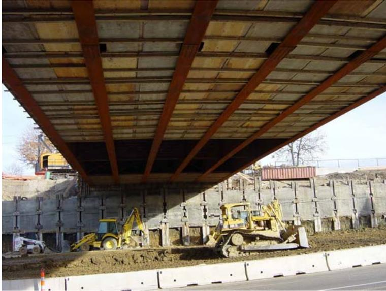
**Figure 3.23. Work platform resting on the bottom flange of the girders over I-235**
