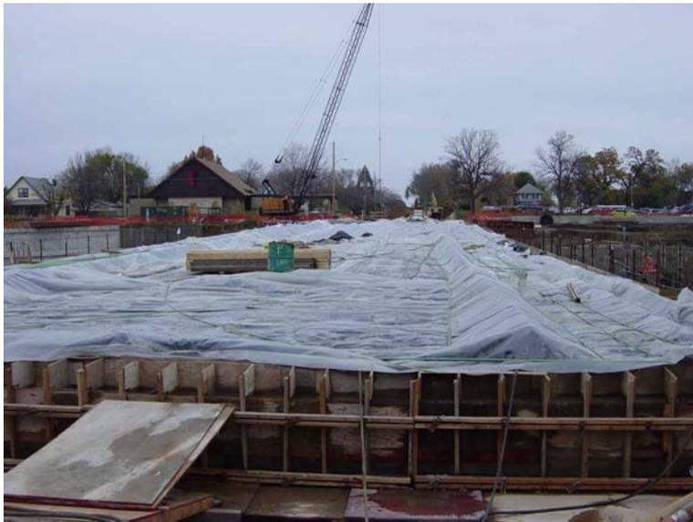
**Figure 3.25. Bridge deck covered after concrete placement**
