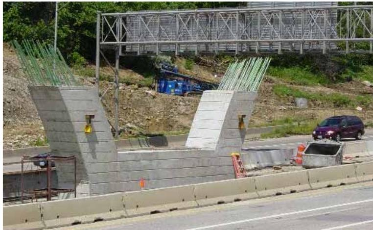
**Figure 3.15. Center pier after formwork was stripped and before reinforcing steel and formwork for the pier cap were constructed**
