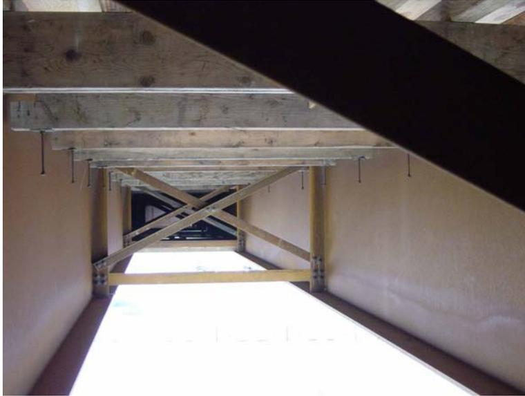
**Figure 3.24. Intermediate cross-frames and deck formwork stringers**
