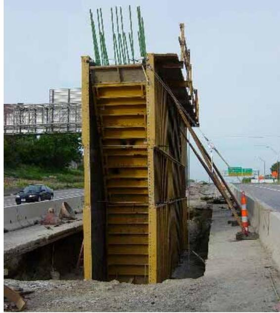
**Figure 3.14. Center pier formwork after assembly and placement**
