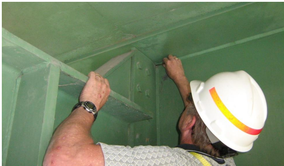
Figure 8. Inspection and measurement (with feeler gage) of pier bearing stiffener fit with top flange of girder.
