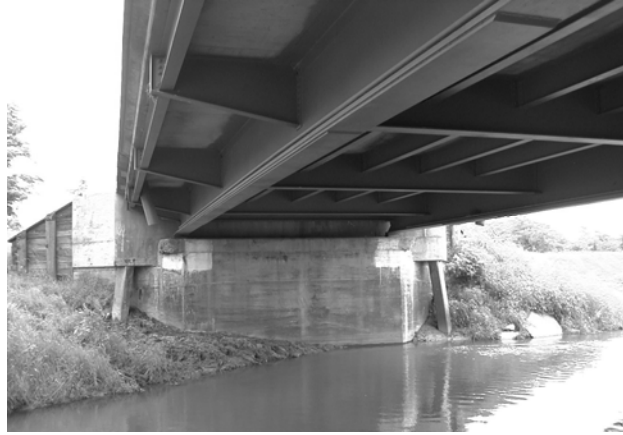
FIGURE 1. Photograph of the main girders of Bridge One.
