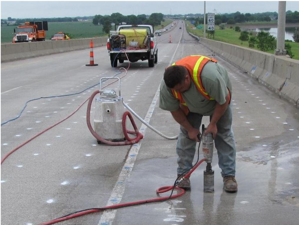
*Figure 2.3. Removal of concrete core sample.*
